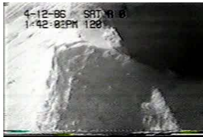
large crushed ice extrusion clearing around the NE face of the caisson
