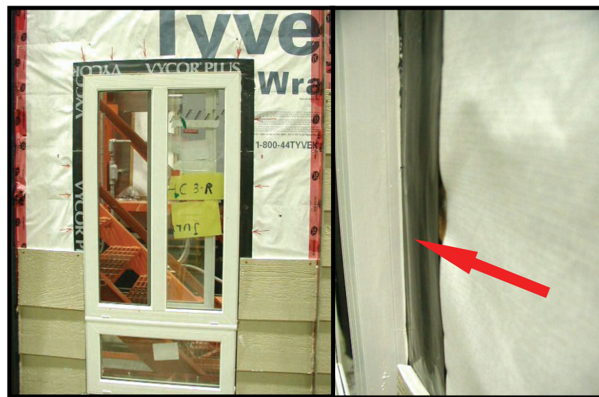
Figure 7-23: Formation of “fish mouths” around the perimeter of the B-side window
