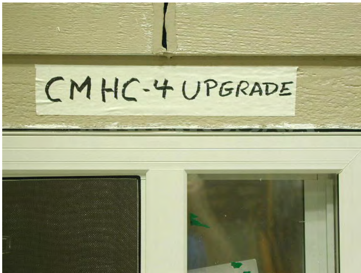
Figure A7-31: Modified Specimen W4. Detail at the window head: no drip cap flashing and gap left open
