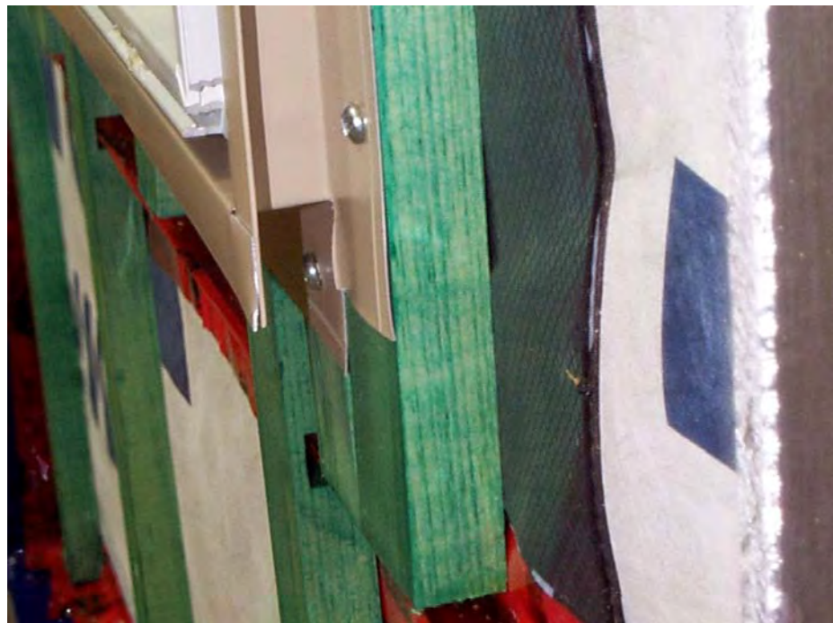
Figure A4-19: View of the bottom corner of the J-trim installation on the furring strips at the sill/jamb corner
