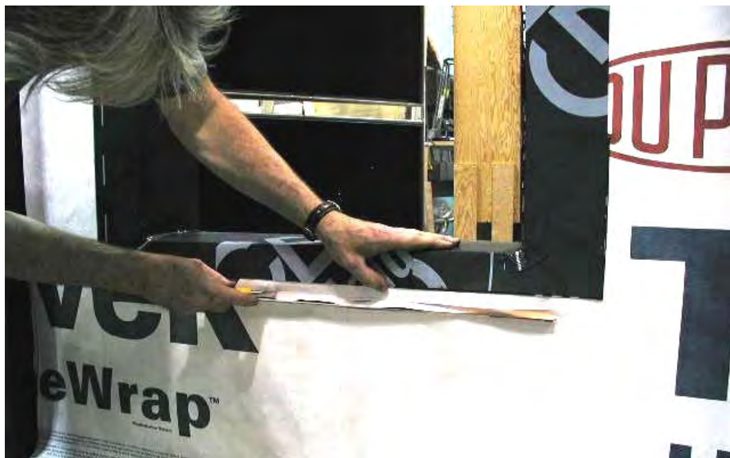
Figure A4-14: Slot for the water collection trough for water running down from the rough sill on the WRB membrane
