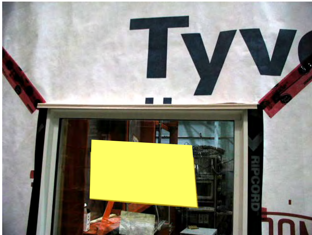
Figure A5-15: Specimen W2 B-side – Water resistive membrane completed
