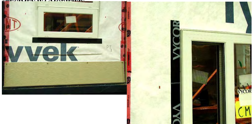
Figure A7-14: Specimen W4 B-side only – Self-adhered membrane installation at sill, and at jambs
