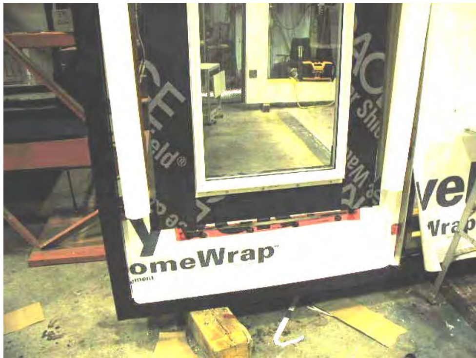
Figure A5-11: Specimen W2 B-side – Installation of the self-adhesive membrane at jambs and head, sealing the flange to the sheathing board
