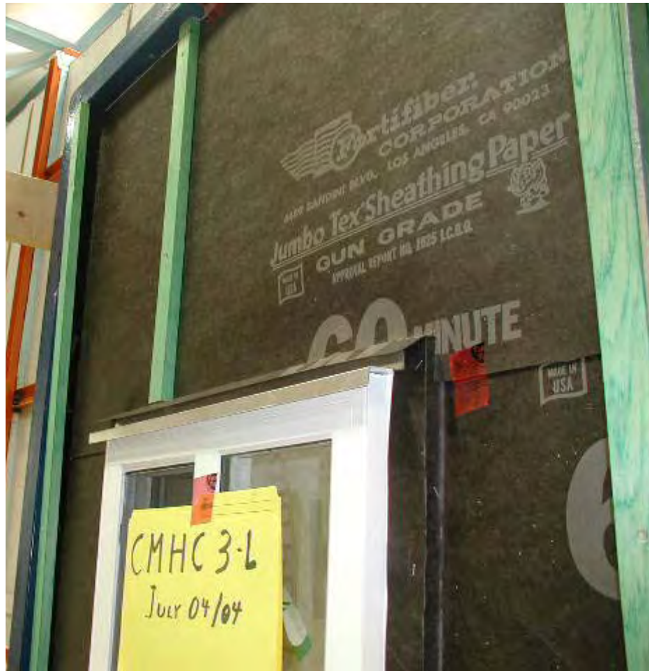
Figure A6-18: Installation of the drip cap flashing and WRB building paper over it (Specimen W3 B side only)
