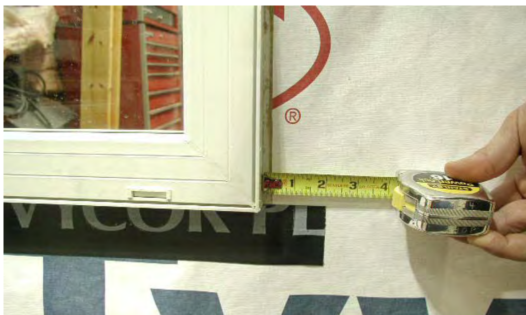
Figure A7-27: Modified Specimen W4 – B-side. Gap left between WRB membrane and window flange, to be covered later by a 50 mm wide strip of flashing membrane
