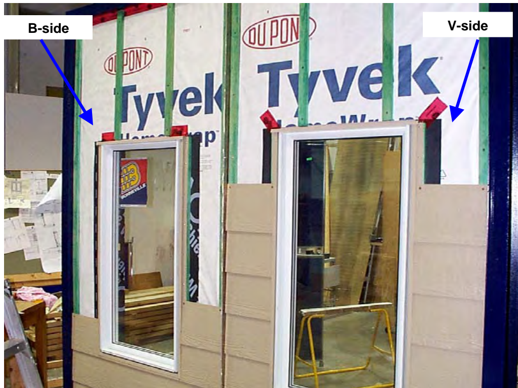
Figure A4-26: Installation of hardboard siding
