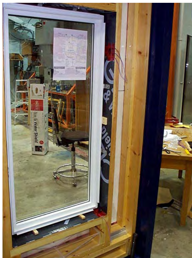
Figure A4-15: View of jamb, sill and head treatment with waterproof membranes at the wall/window interface
