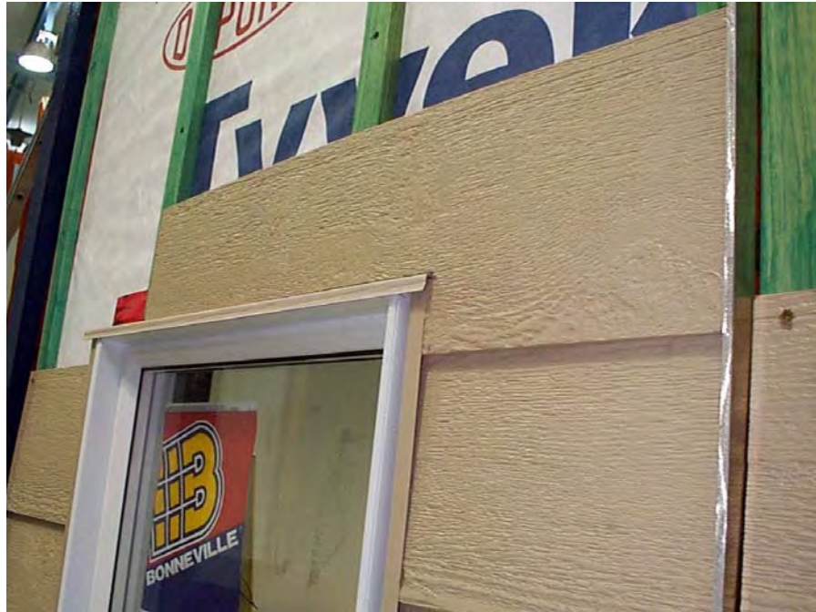
Figure A4-23: Upper corner of the wall/window interface detail
