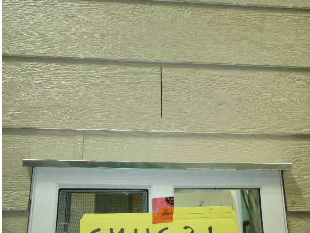
Figure A6-23: Saw cut (3mm thick by 150 mm long) in the hardboard siding, acting as a deficiency potentially allowing water ingress above the window
