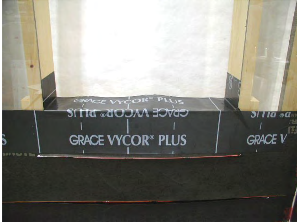
Figure A6-12: Specimen W3 B-side – Waterproof membrane installed, lapping down over the first course of building paper by 150-mm
