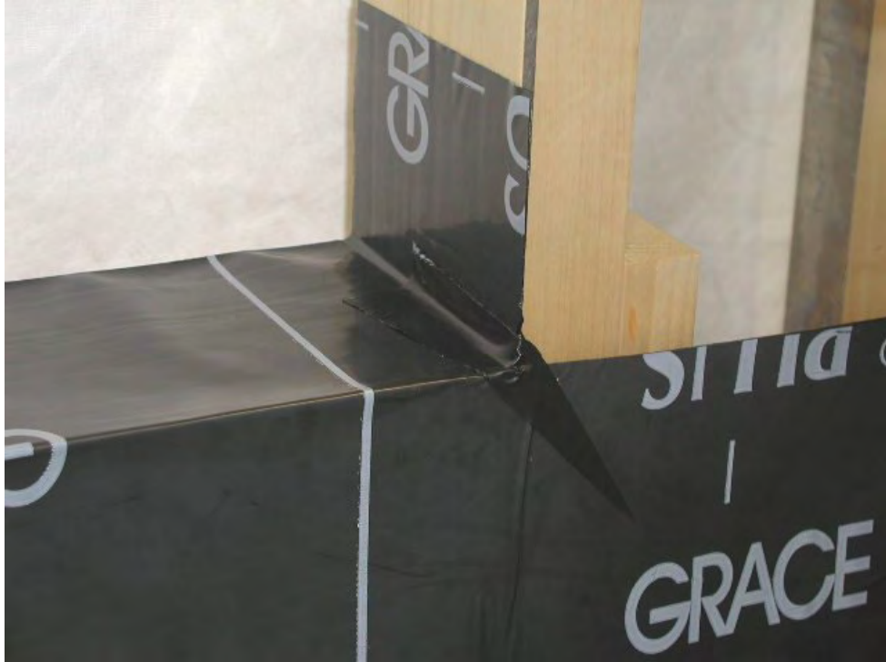
Figure A6-11: Specimen W3 B-side – Installation of the waterproof membrane onto the subsill, over the sheathing board below and up rough jambs (150-mm). Corner piece of waterproofing membrane also applied.
