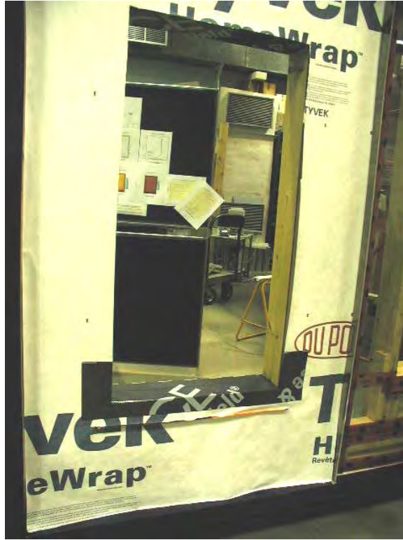
Figure A4-12: Protection of the rough sill with waterproof membrane
