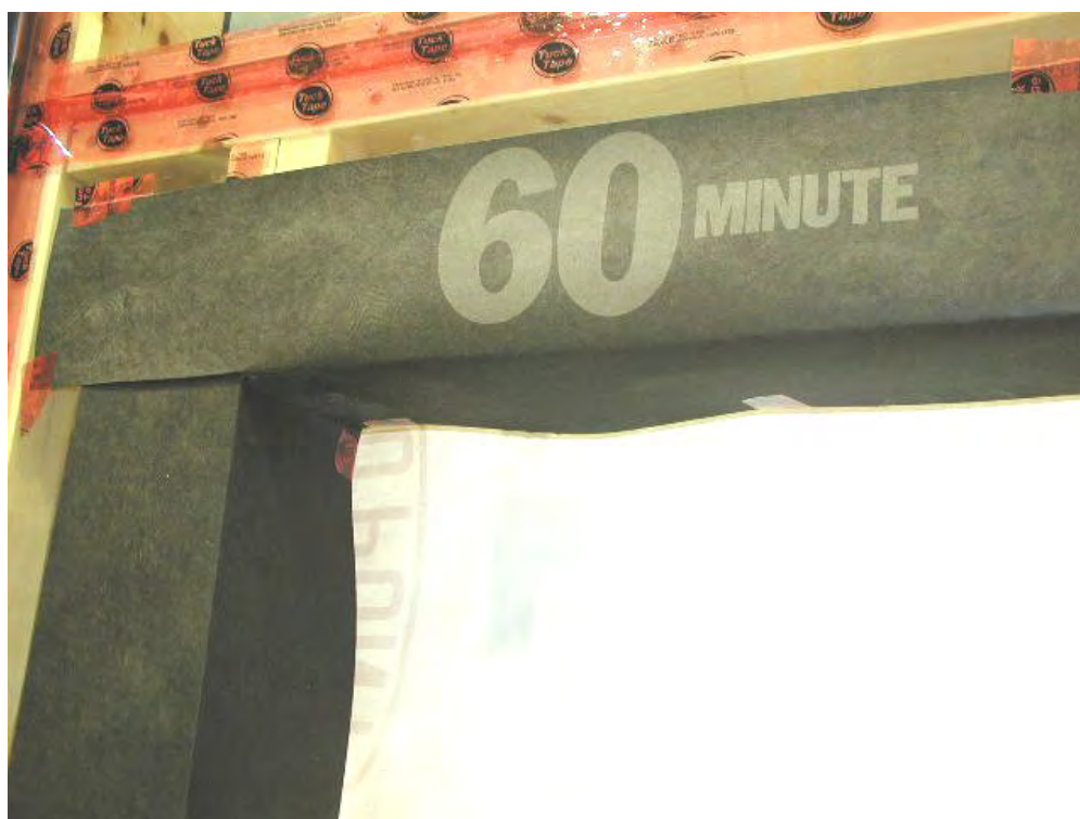
Figure A6-15: Specimen W3 B-side – Installation of strips of 60 minute building paper at rough head
