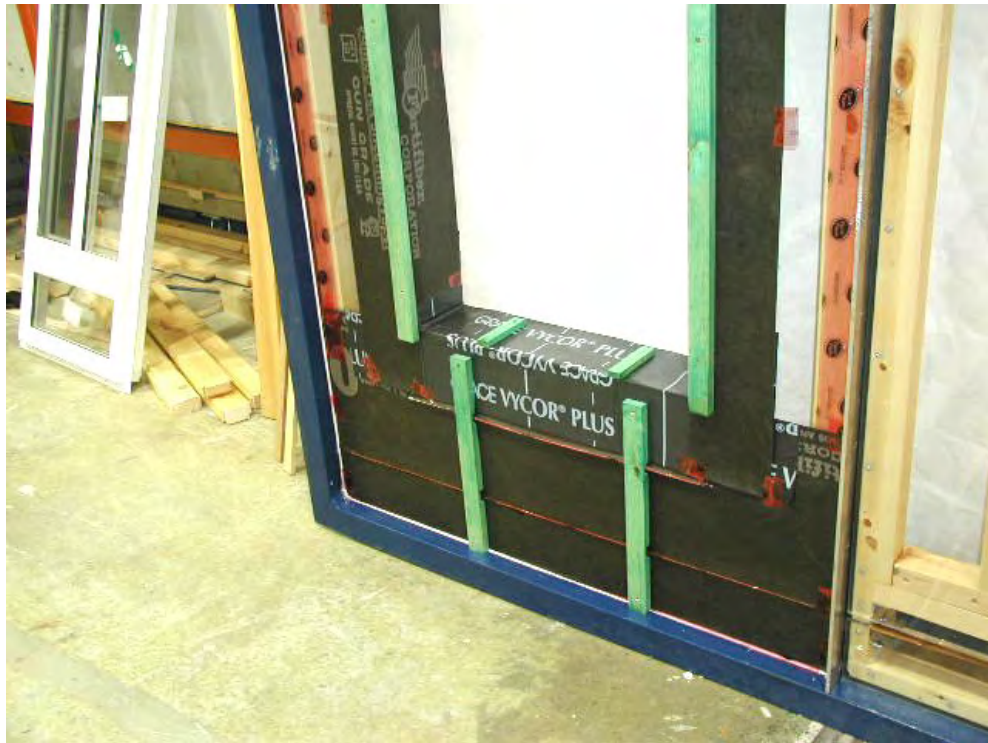
Figure A6-16: Specimen W3 B-side – Installation of the furring strips prior to window installation (Left side of Specimen only)
