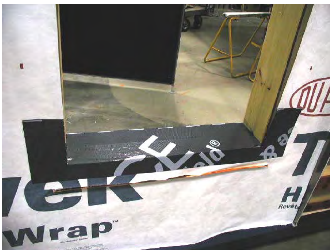
Figure A4-11: Installation of flashing membrane onto the rough sill
