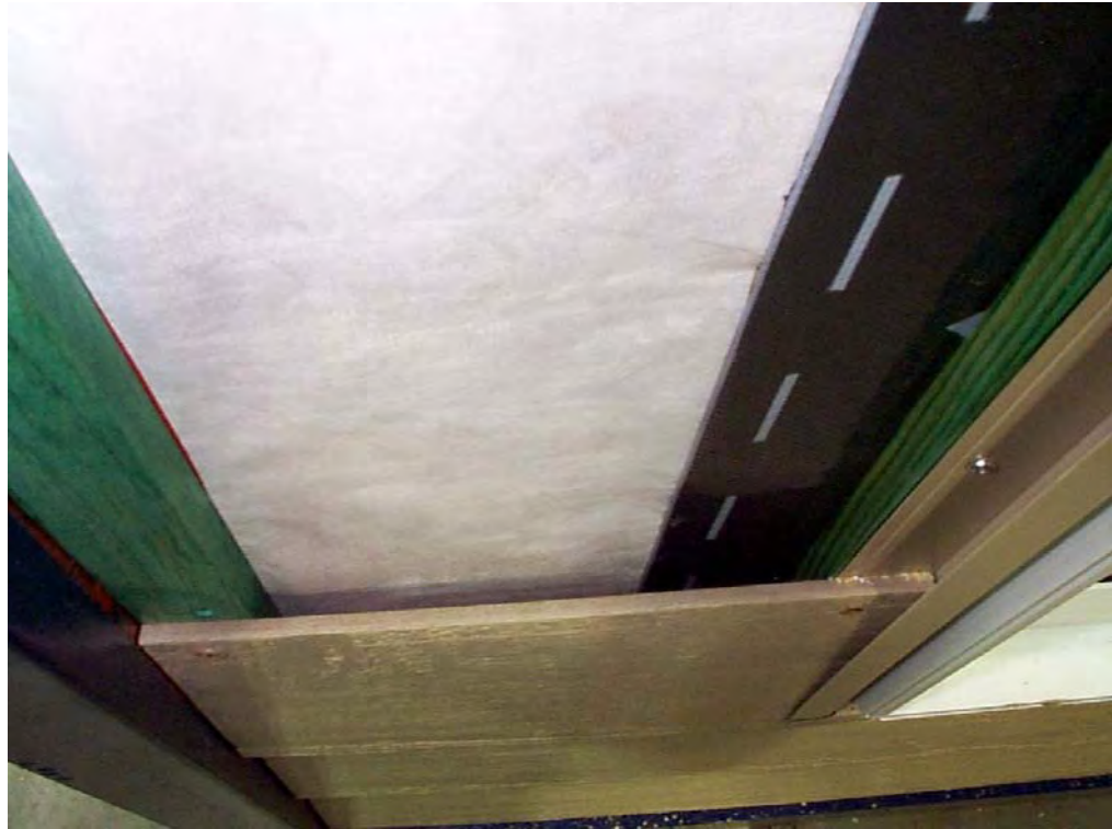
Figure A4-27: Descending view of the air space behind the siding
