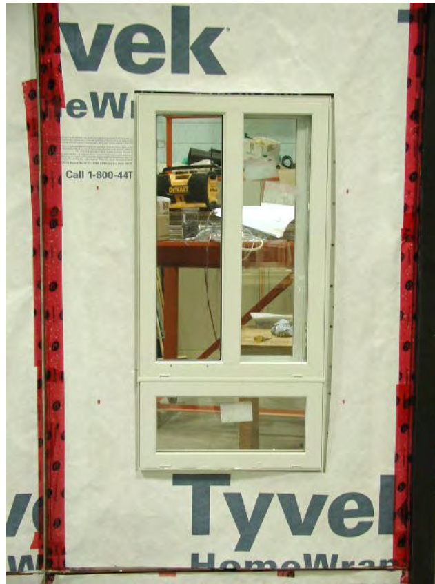
Figure A7-24: Modified Specimen W4 V-side – Installation of WRB membrane
