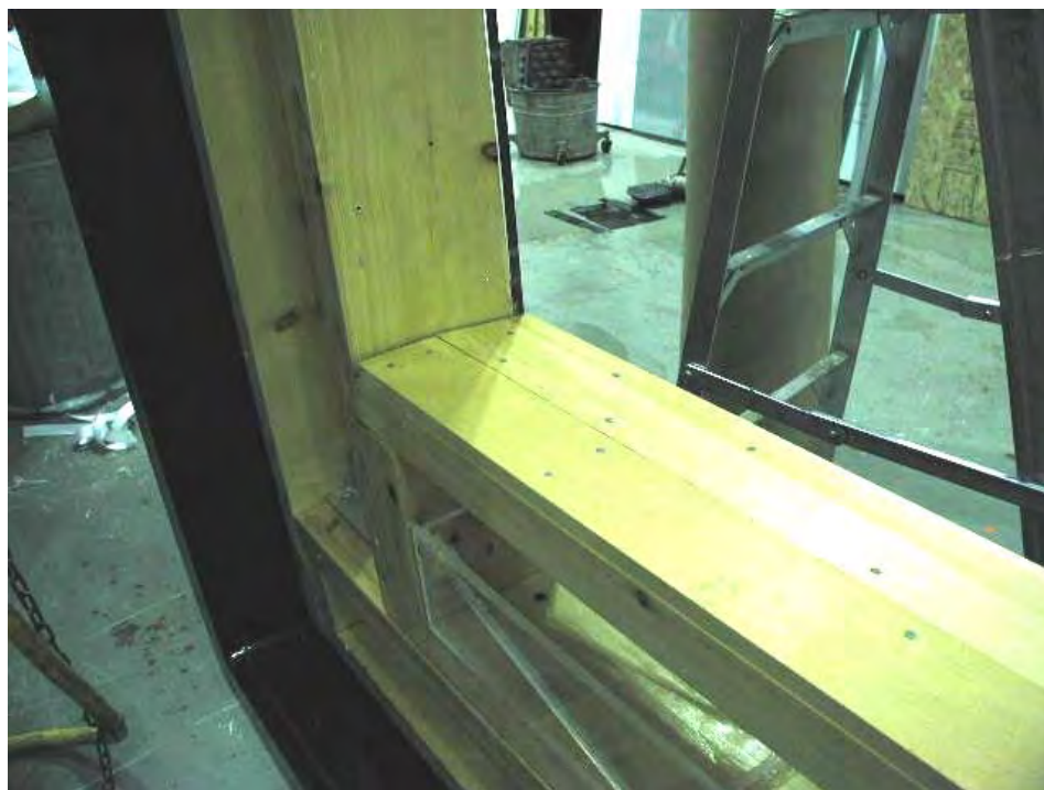
Figure A4-10: Sloped rough sill
