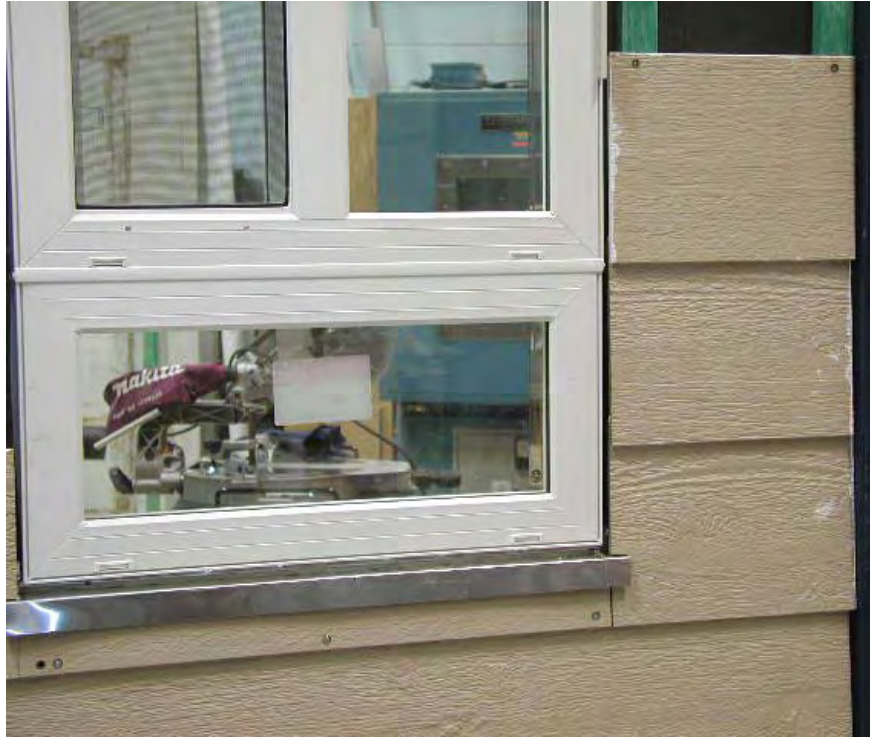
Figure A6-21: Siding installation. 10 mm gap left at the jambs and sill for a backer rod and sealant
