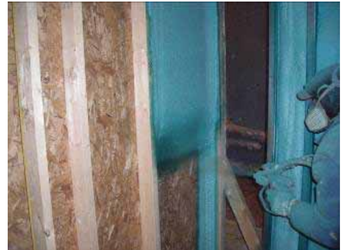
Wall insulation example Picture frame technique
