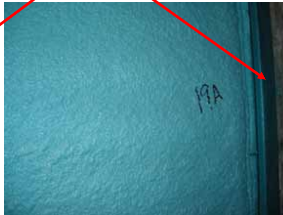
Steel foam interface Cavity side of stud
