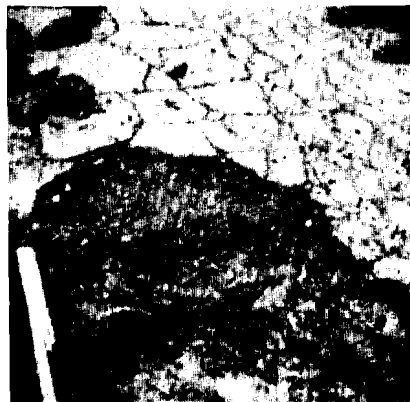
Fig. 5. On digging up a superficially dry, damaged place, seepage water is found emerging from a roadbed.
