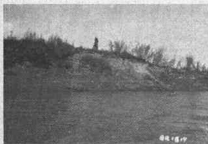
Fig. 1. Natural exposure on bank of stream—thawing occurring accompanied by slumping.
