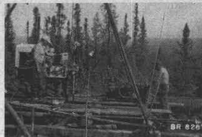
Fig. 8. Standard diamond drill set-up for coring frozen soil and bedrock.
