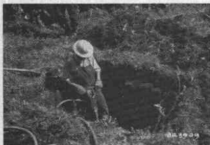
Fig. 6. Starting test pit using air-powered jack hammer.
