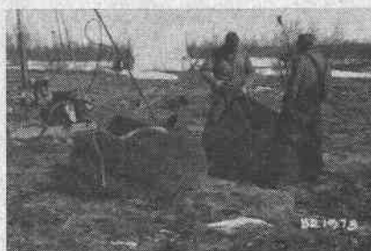
Fig. 10. Filling 300-gallon capacity canvas bags for water supply at drill site.
