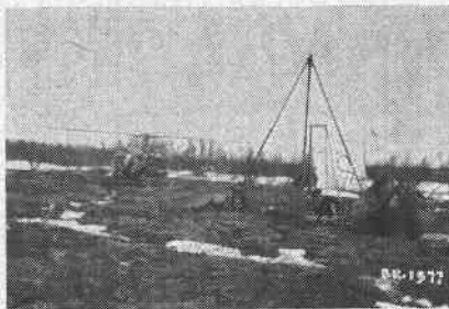
Fig. 7. Special light core drill moved to drill site by helicopter. Tent in background is used for soil sampling and photographing frozen cores.
