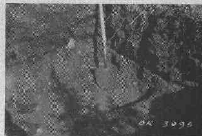
Fig. 3. Test pit excavation by natural thawing. Removing thawed material from test pit excavated in gravel.
