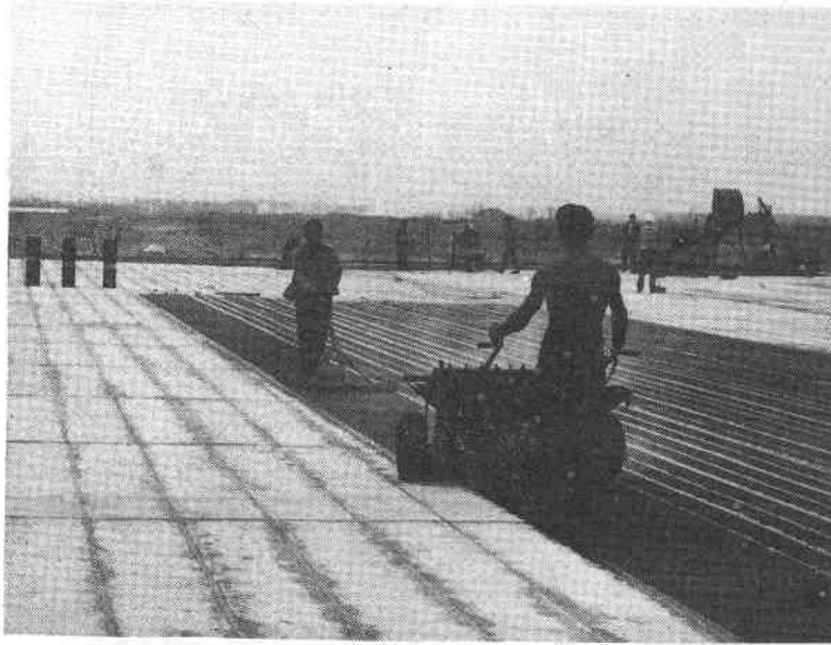
Figure 5 Machine laying of felts by the shingle method. Usually better than hand mopping but still leaves direct path from roofing surface to substrate if adhesion is poor or wrinkles occur between plies.
