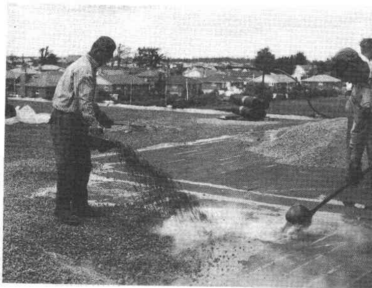
Figure 6 Top pouring of bitumen with gravel spread by hand. Uniform coating is unlikely and possibility of skipped areas great.
