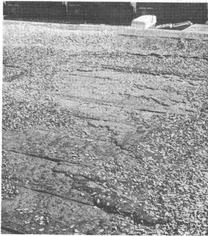
Figure 7 Result of poor gravel surfacing and wind action. Bitumen and felts are completely unprotected.
