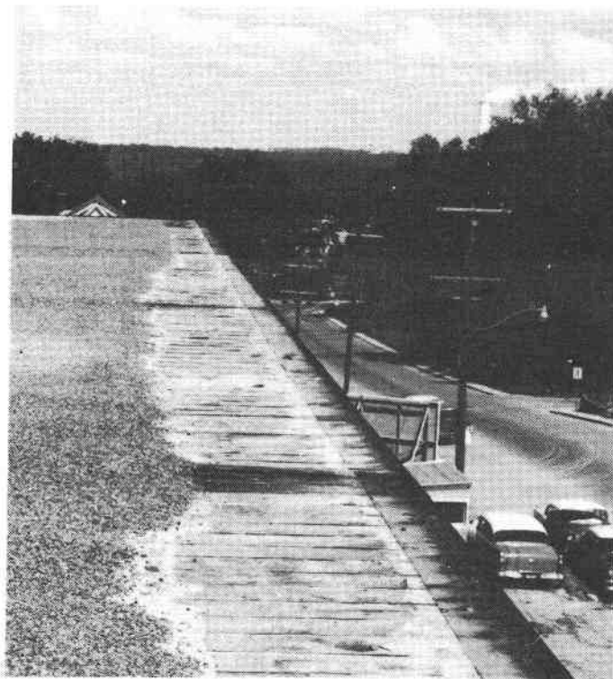
Figure 8 Because of poor flashing design, work at roof perimeter has been left for completion at a later time. Felts are unprotected and will be very much deteriorated before the job is finished off.
