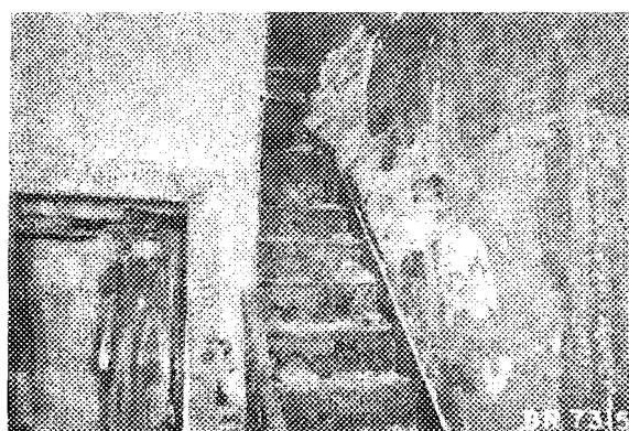
Fig. 14 Open front staircase where heat and gases extended to second floor.
