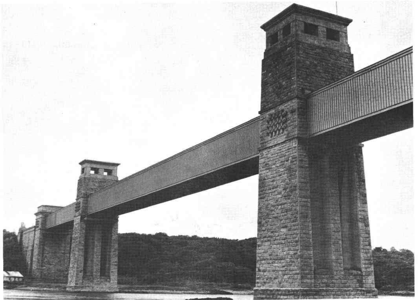
FIGURE 1: The Britannia Bridge of Stephenson and Fairbairn, 1849, perhaps the first large stressed skin structure (courtesy London Midland Region, British Railway).
