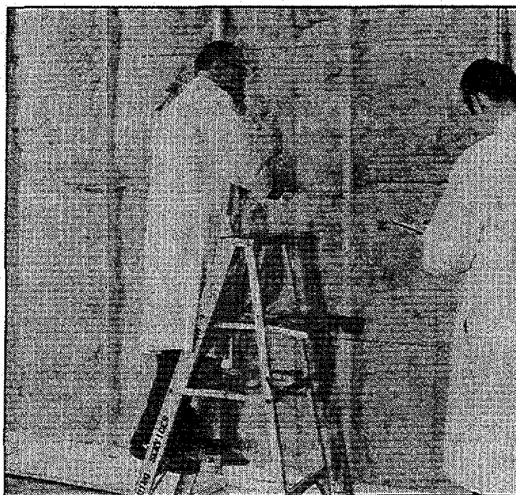
Early IRC research on insulation revealed that the fit of insulation in stud spaces of wood-frame walls and the stability of the insulation in place can affect the performance of the wall.
