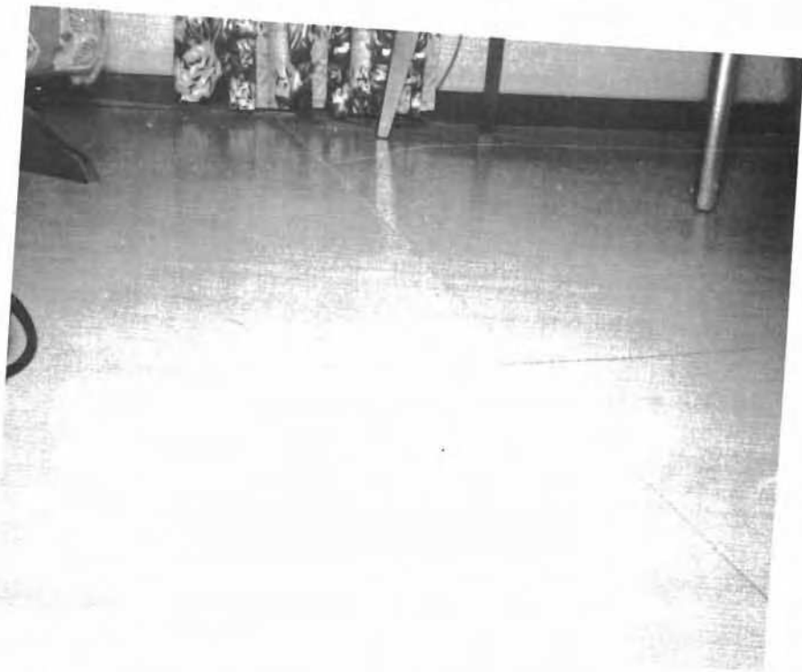
Figure 7 Separation of plywood flooring sheets -- Mark II House.
