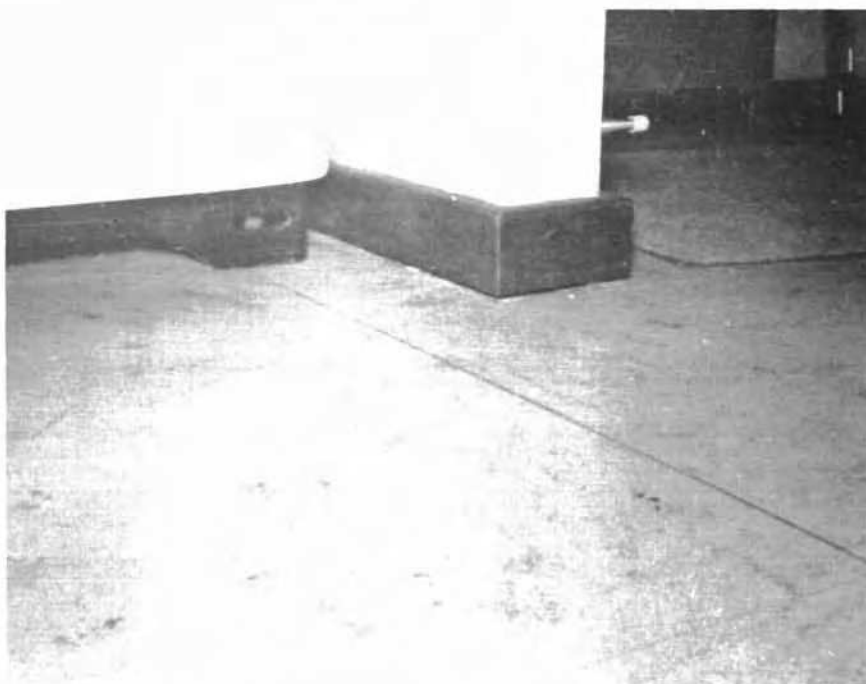
Figure 8 Separation between base of wall and floor -- Mark II House.
