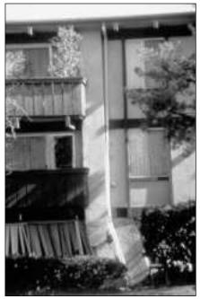
Figure 2. Excessive deformation of a weak first storey in an apartment building, Northridge earthquake 1994. In another part of the building the ground floor collapsed completely.
