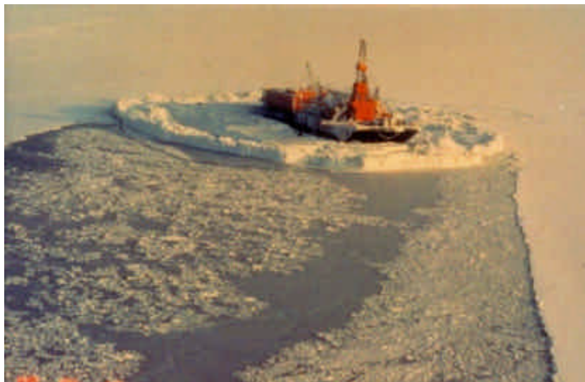
Figure 5.6: Representative views of pack ice moving past the SSDC and its grounded ice rubble annulus (and its flooded ice berm) in winter. These photos were taken when the SSDC was deployed on a sand berm at locations in the moving pack ice zone the Canadian Beaufort Sea.
