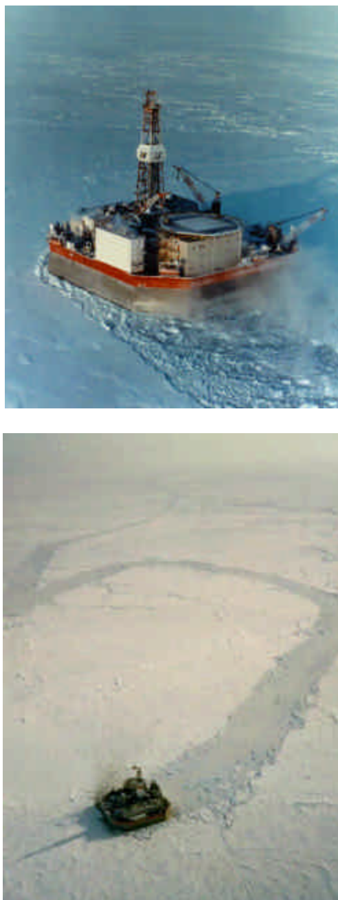
Figure 5.7: Representative views of moving pack ice around the Molikpaq in both thin and thick ice conditions showing the down-drift wakes that were often seen behind the structure.
