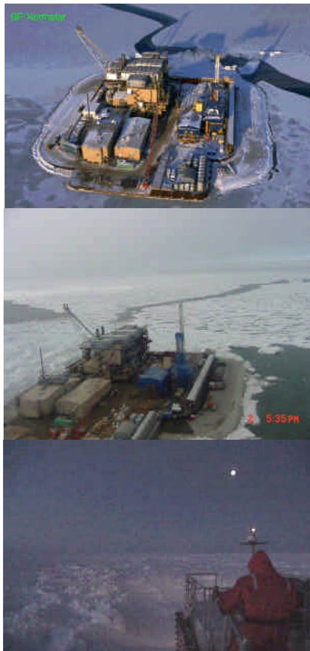
Figure 5.16: Typical views of the Northstar production island during freeze-up and break-up ice situations (top and middle photos). In winter, the ice cover and grounded rubble around this platform is stable. The lower photo shows an ARKTOS craft moving over nearby rough ice in winter, during a training exercise for a driver. The ARKTOS craft has been selected as the primary means of evacuation in certain ice and emergency situations.
