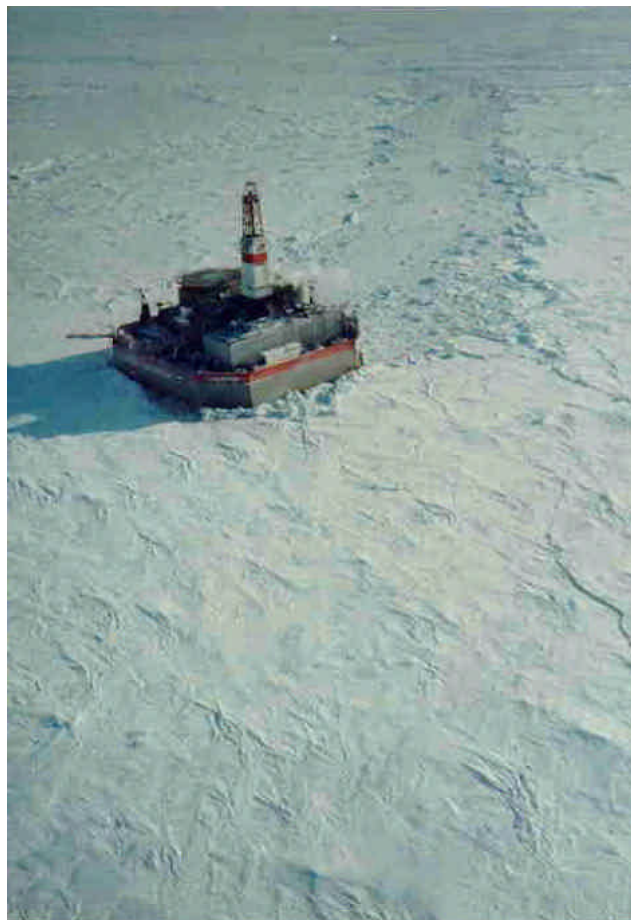
Figure 6.1: Photograph showing ice action on the updrift sides of the Molikpaq in moving pack ice, and the brash ice wake behind it.
