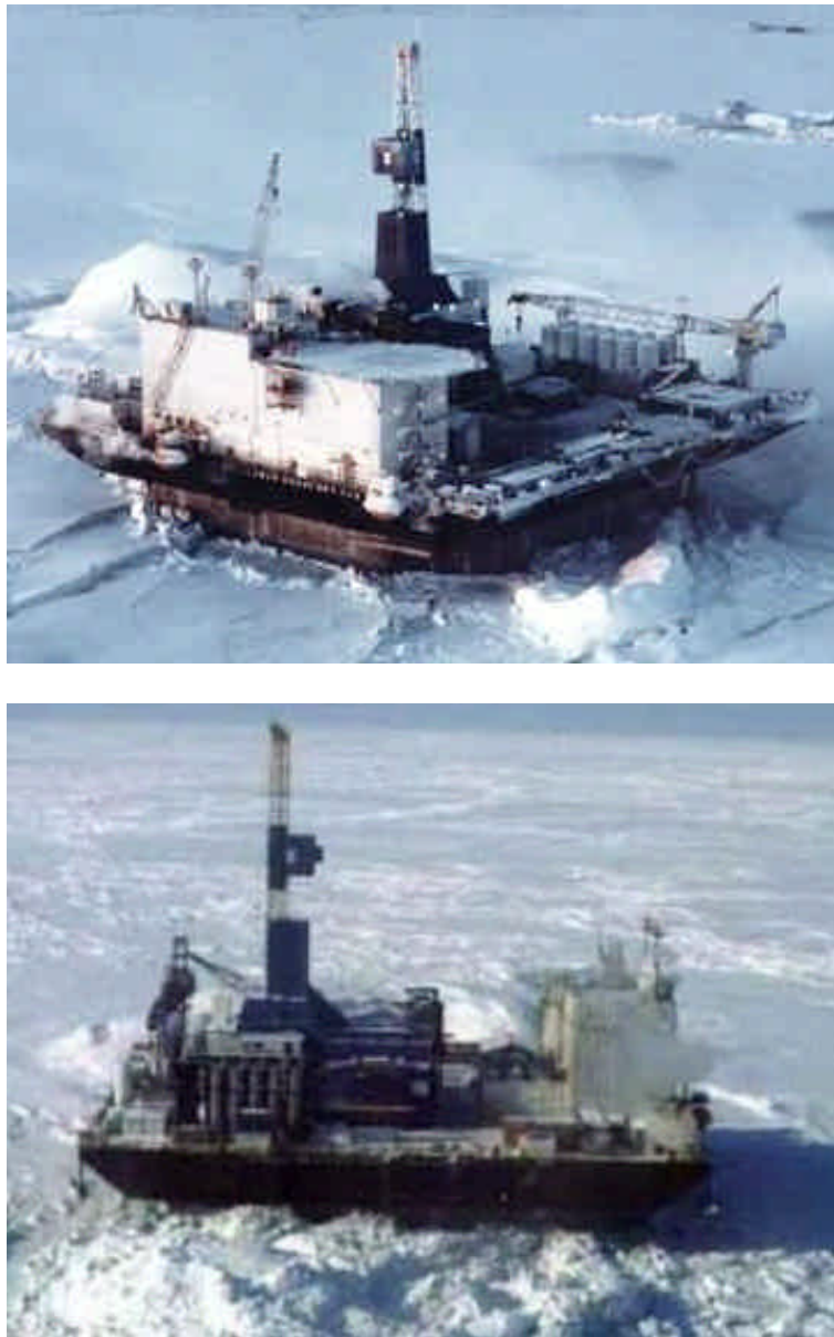
Figure 5.15: Typical views of the CIDS in ice. The upper photo shows the drilling unit in thin ice during freeze-up, with a protective spray ice berm under construction. The lower photo shows the structure in more stable winter landfast ice conditions.
