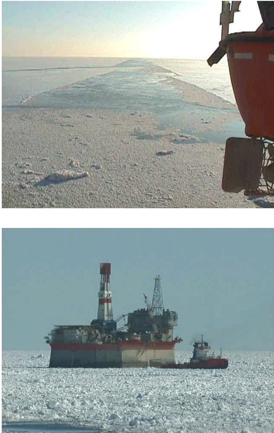
Figure 6.6: Downdrift wakes can sometimes be quite open (upper - in thin moving ice) and at other times full of brash and broken ice fragments (lower - in small floes). Although these photos were taken around the Molikpaq off Sakhalin Island, observations in the Beaufort Sea were similar.
