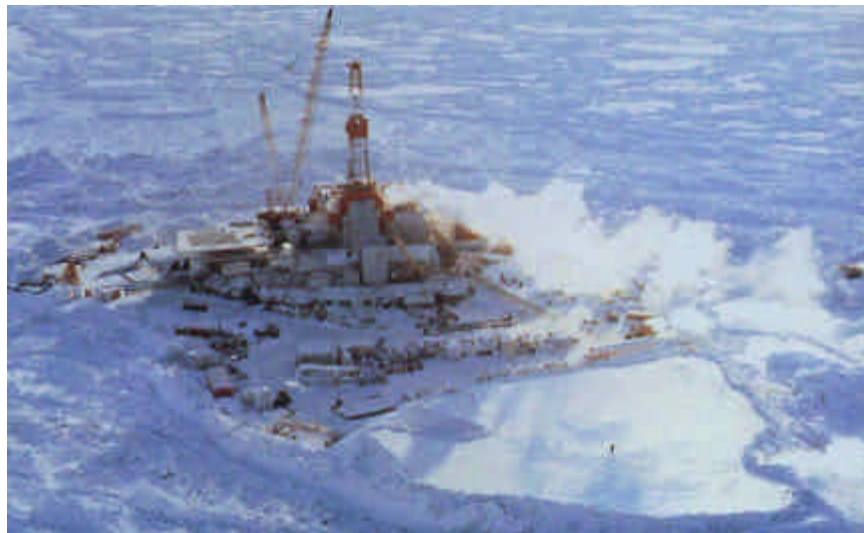
Figure 5.2: Representative views of the type of stable landfast ice conditions that were seen at the Tarsiut CRI during the winter period, including the grounded ice rubble annulus around it, and its relief well ice pad.
