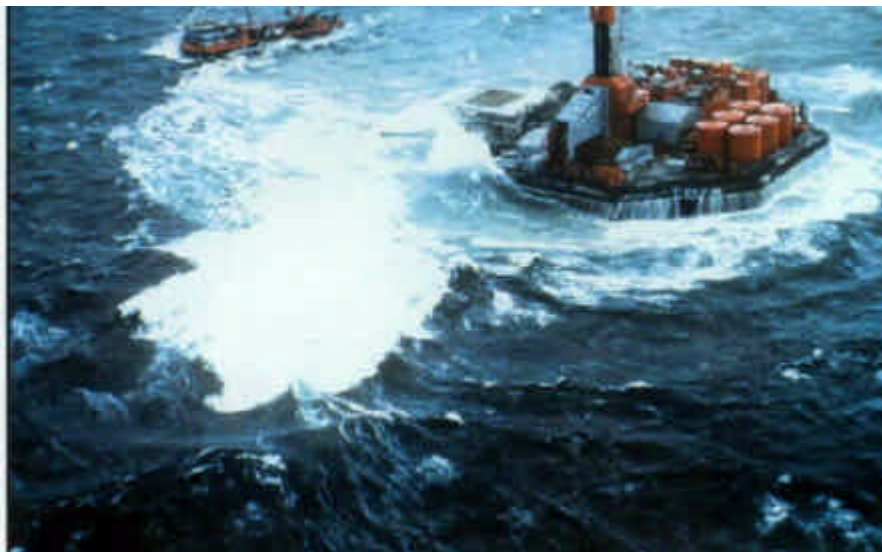
Figure 5.3: Representative views of the type of thin moving ice conditions that were seen around the Tarsiut CRI during freeze-up (upper aerial photo), and in storm waves during the open water season (lower).
