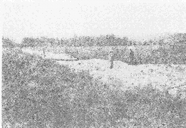
Plate 13 Thaw Settlement of Road Passing Through Area of Ice-Rich Soil (Great Khingan Range)
