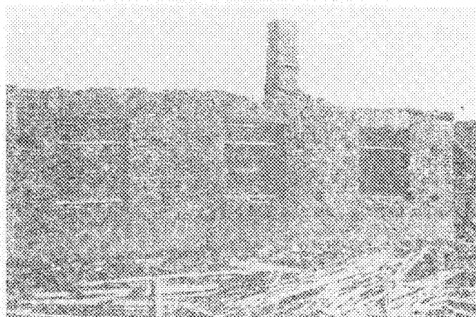
Plate 9 Building Damaged by Frost Heaving
