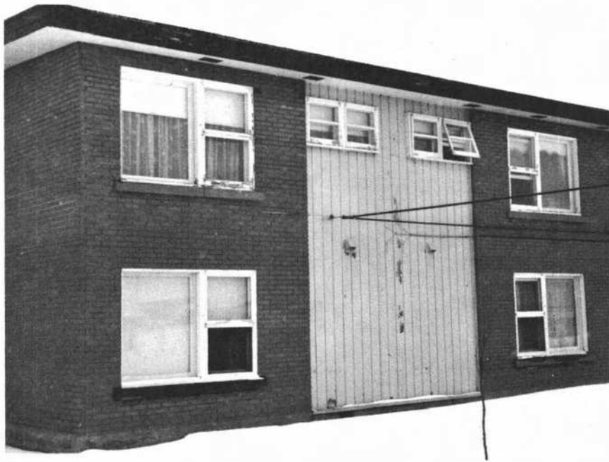
Figure 9 Rear of buildings at Place St. Louis, Boucherville, showing paint peeling at centre of panel and on sash
