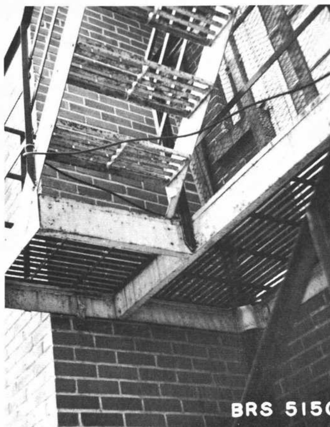
Figure 12 Exterior metal stairways at Boulevard Pie IX, Montreal, showing rusting
