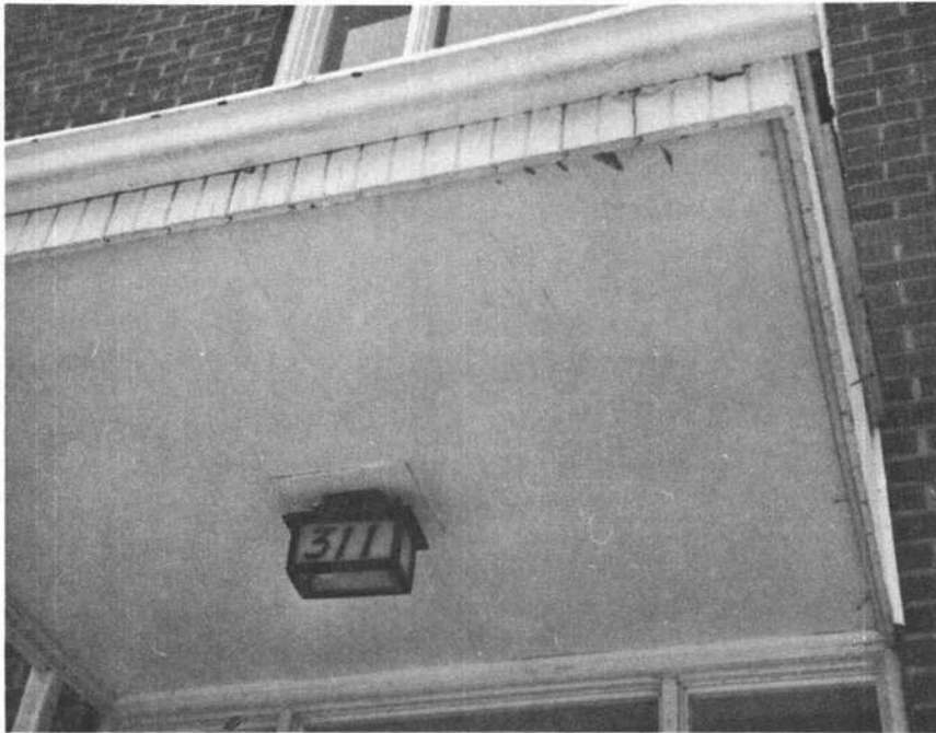
Figure 5 Plywood ceiling of door canopy at Cumberland Court, Cornwall, showing cracks and peeling at outer edges
