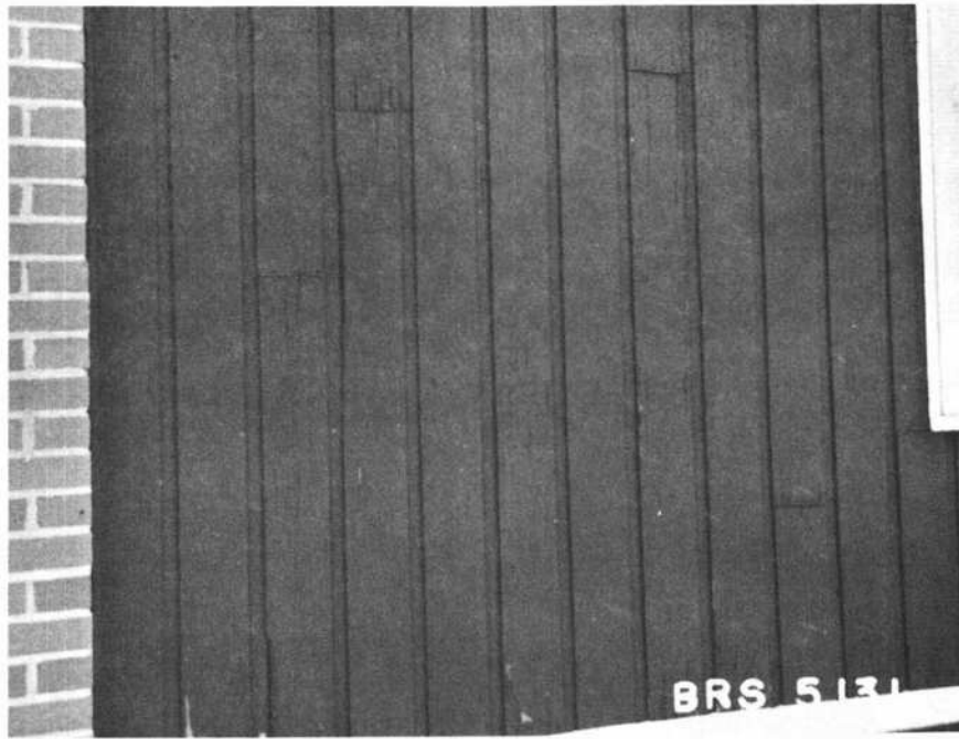
Figure 3 End panels of buildings at Brookdale Terrace, Cornwall, showing poor wood used in construction
