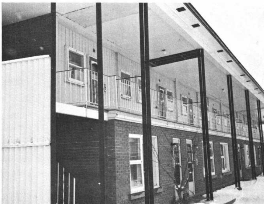
Figure 8 Protected facing on row housing at Place St. Louis, Boucherville
