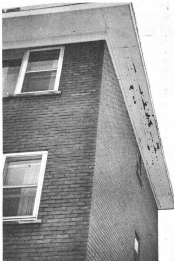
Figure 7 Paint peeling on vented soffits at Cloverdale Park, Pierrefonds
