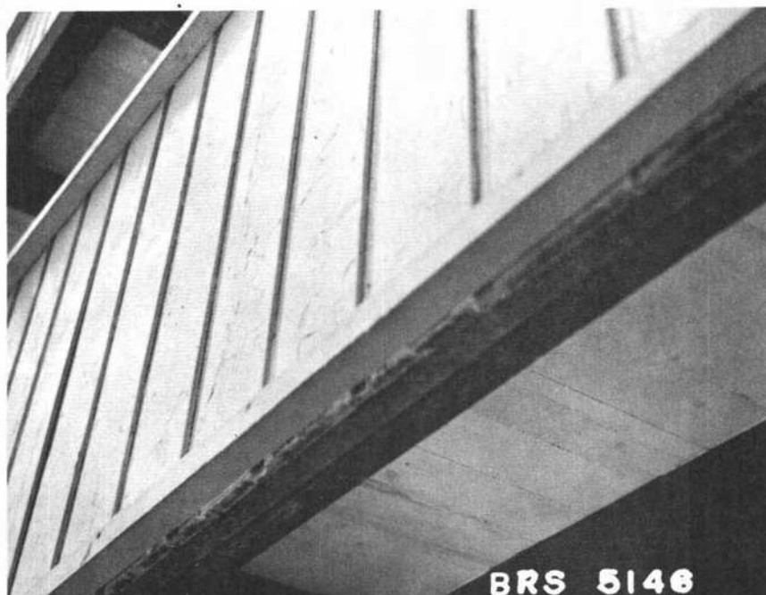
Figure 11 Irregular removal of old paint on balcony at Boulevard Pie IX, Montreal
