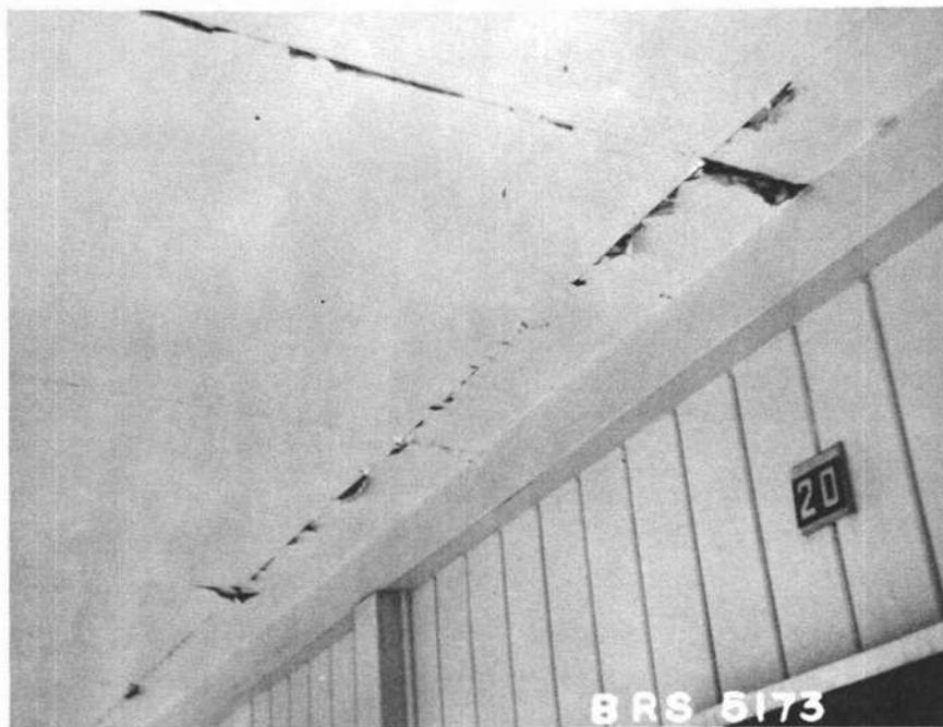
Figure 10 Porch ceiling at Place St. Louis, Boucherville, showing buckled plywood and peeling paint
