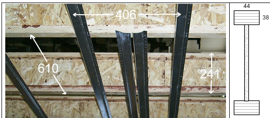
Figure 1: View and cross section of 241 mm deep I-joist. The joists were spaced 610 mm o.c. in this case.
