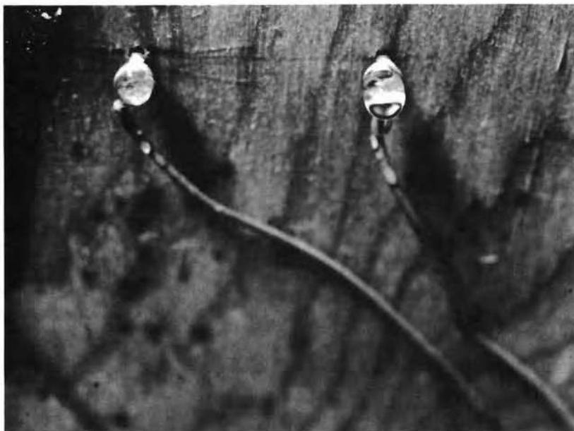
Figure 22 Panel D, space 11. Fungus on wet roof deck.
