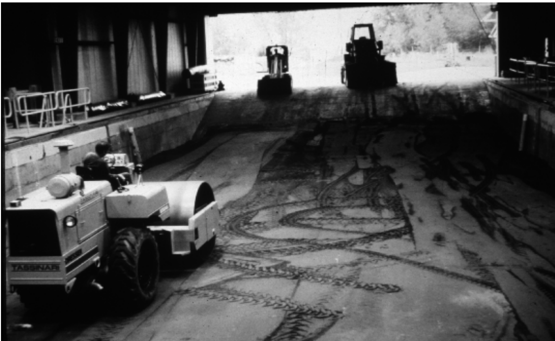
FIGURE 11: Typical Full-size Construction Equipment for Test Section Construction.
