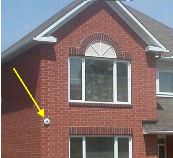
Figure 6 - Pyranometer Location on Reference House South Façade
