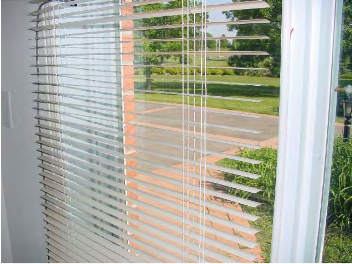
Figure 5 - The Benchmark shading configuration - Venetian blinds in the down and horizontal position
