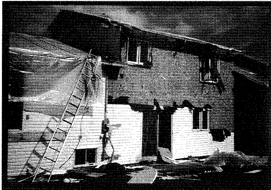
Figure 8 Siding stripped from west (windward) wall of house in Figure 7.
