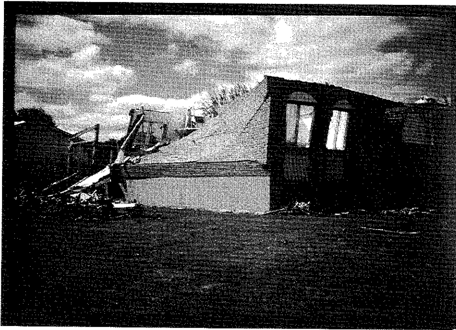
Figure 11 Brick wall collapse showing progressive failure once roof is gone and connection to west (windward) wall is lost.
