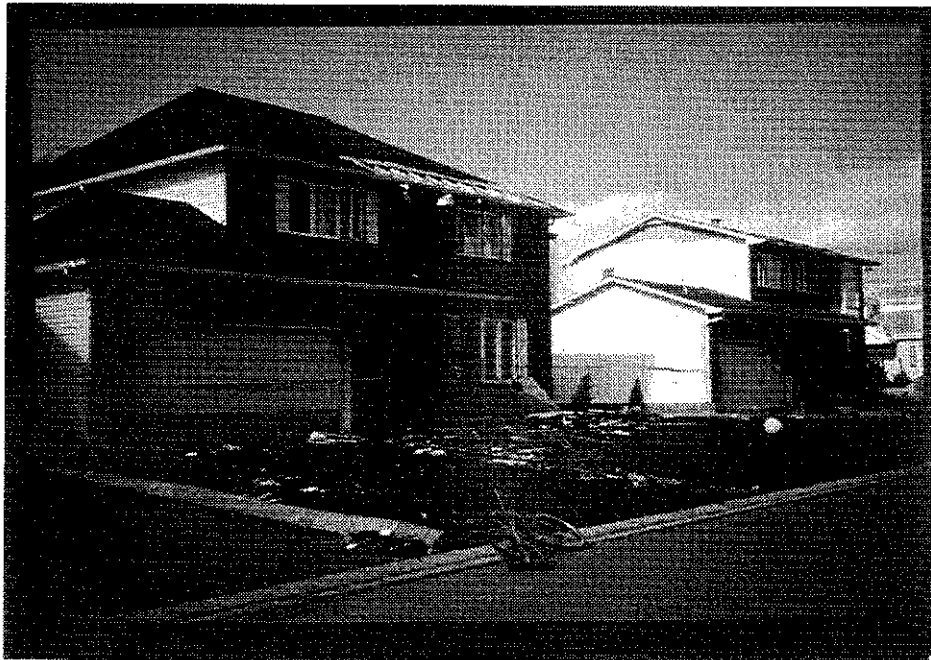
Figure 3 Wind damage limited to eave area at southern end of hip roof.
