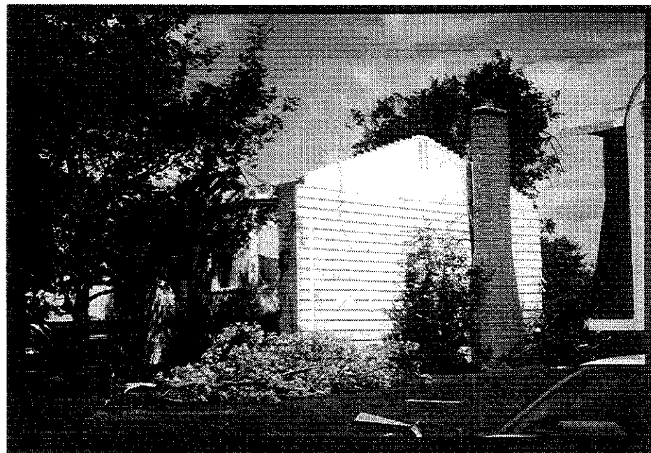
Figure 9 Gable roof lifted off single-storey house, showing south wall, roughly parallel to tornado path.
