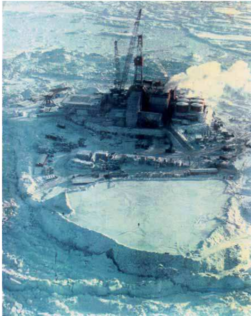
Figure 16: Overhead view of Tarsiut Island in the Beaufort Sea. Note the large ice pad at the bottom of the photograph. This was built as a pad for relief well drilling, if required.
