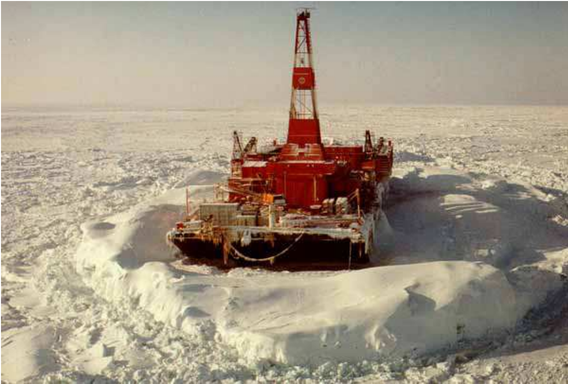
Figure 18: SSCC at the Kogyuk site with a protective spray ice pad.
