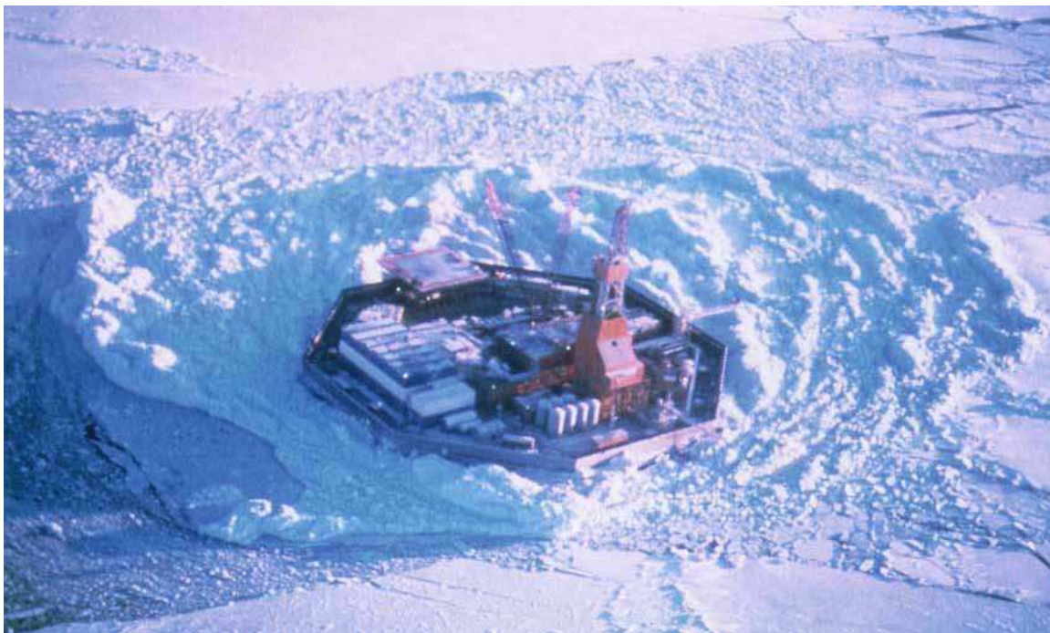
Figure 20: Esso Caisson Retained Island (CRI) with a grounded rubble field.
