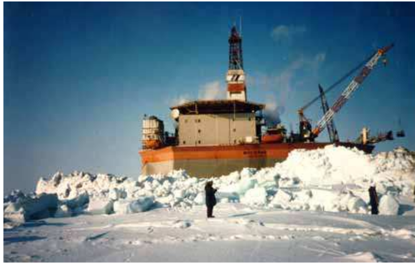
Figure 22: Photograph of the Molikpaq with grounded rubble surrounding it.
