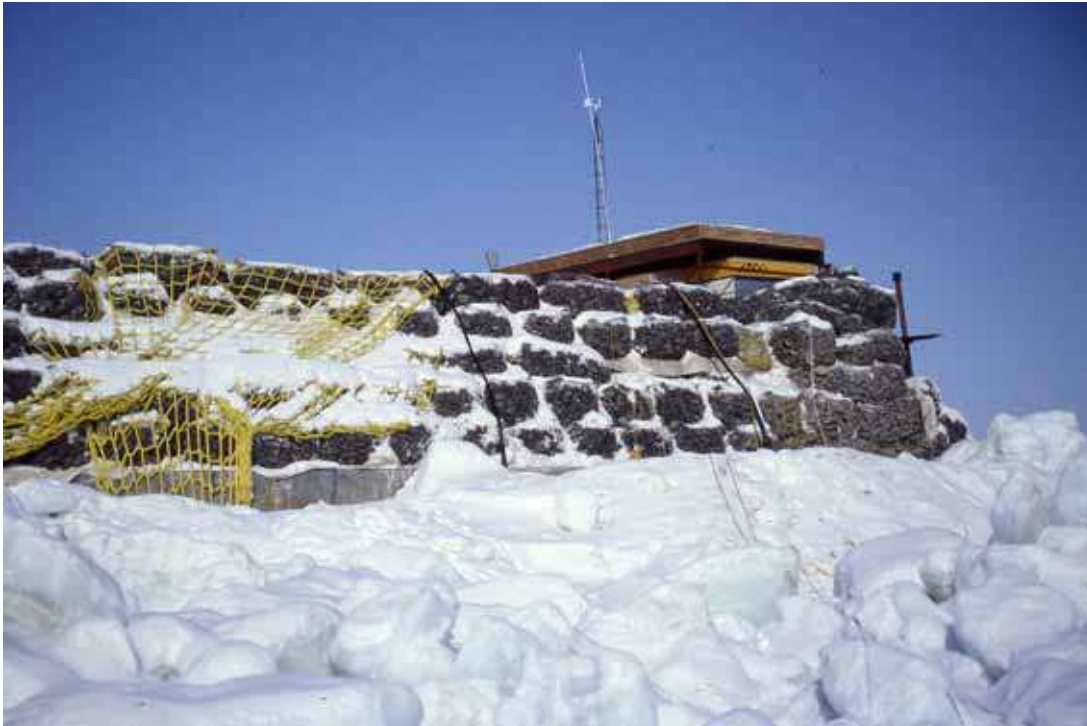
Figure 17: Photograph of the Tarsiut caisson showing the rock-filled gabions that were used to prevent wave overtopping during the summer months.
