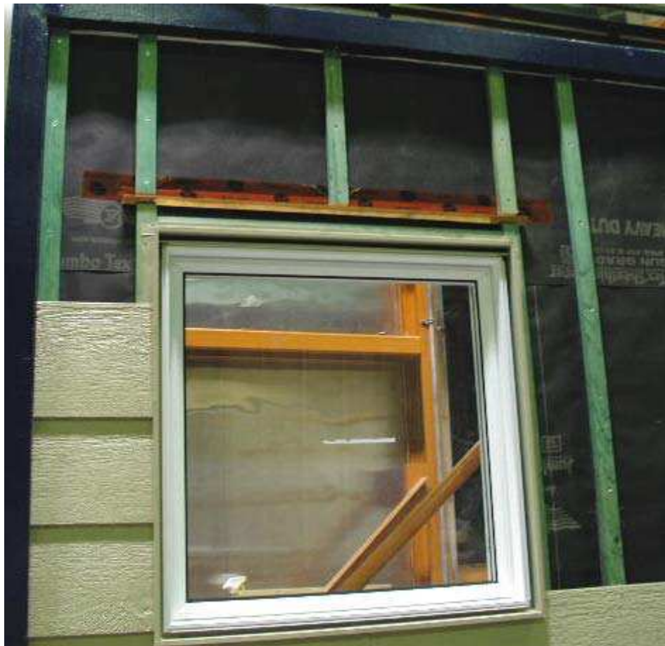
Figure A4.8 Specimen No.16. Detailing around the window of, showing the furring strips, J-trim and deflector at head
