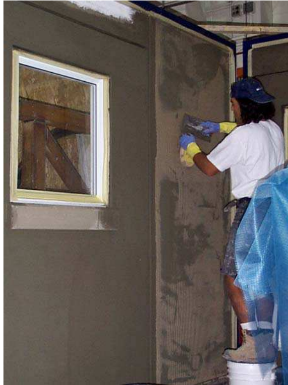
Figure 2.60. Wall No. 8. Application of base-coat and mesh
