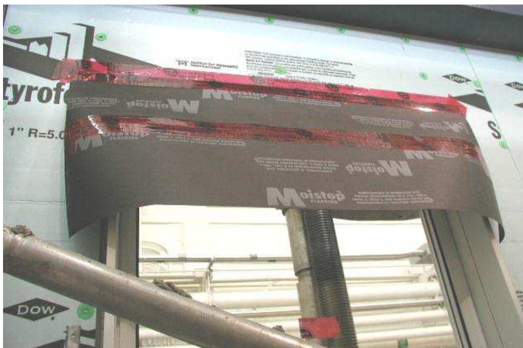
Figure A3.2 Installation of the flashing membrane at the window head of specimen No. 11
