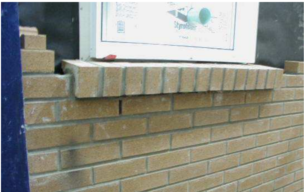
Figure A3.11 Rowlock window sill for specimen No. 12
