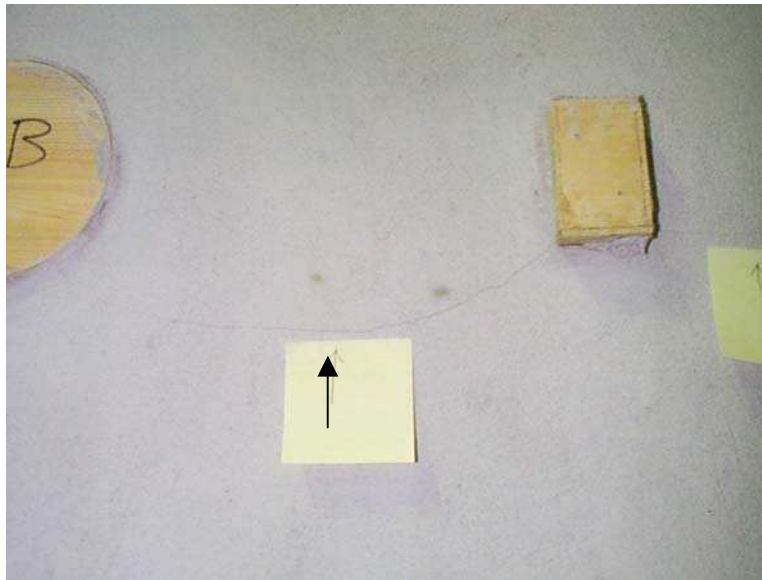
Figure 1.44. Crack between duct and electrical outlet openings (see arrow on sticker)
