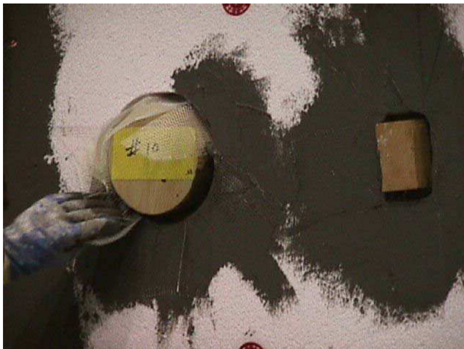
Figure 2.72. Wall No. 10. Backwrapping of penetrations
