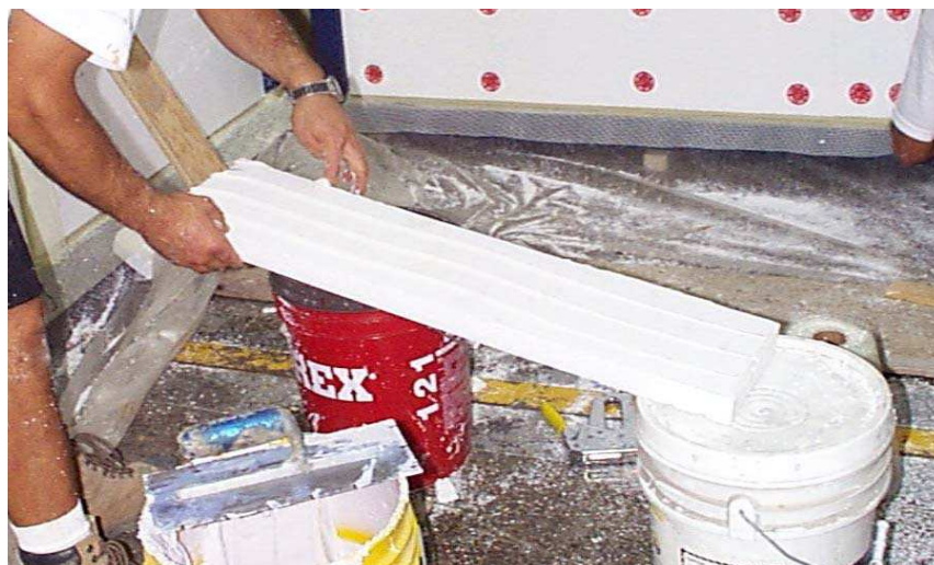
Figure 2.47. Wall No. 6. Application of adhesive to the back of the EPS insulation
