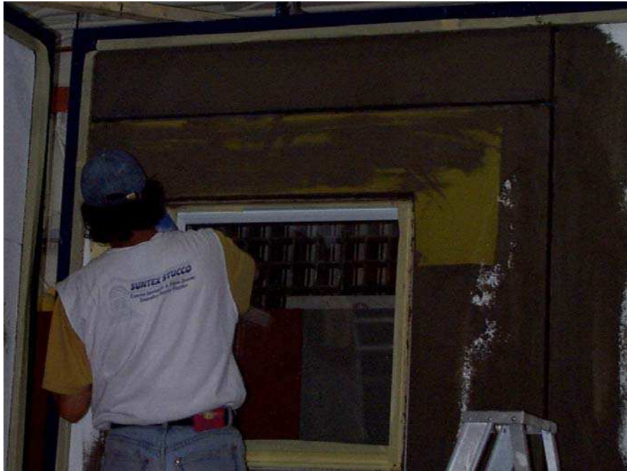
Figure 2.73. Wall No. 10. Installation of base-coat and mesh
