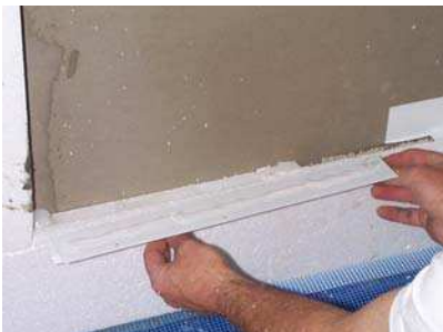
Figure 2.64. Wall No. 9. Drainage system components
