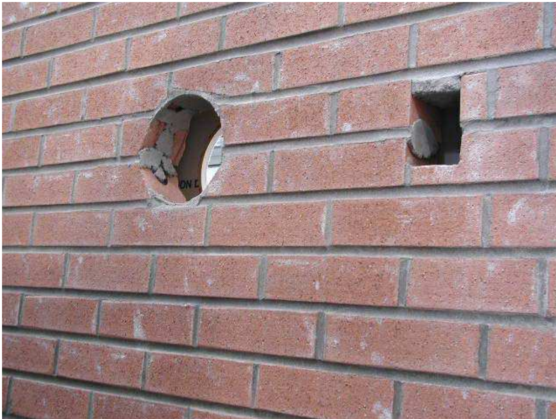
Figure A3.21 Forms were removed for the installation of the ventilation duct and electrical outlet
