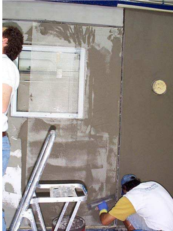
Figure 2.56. Wall No. 7. Application of base-coat and mesh
