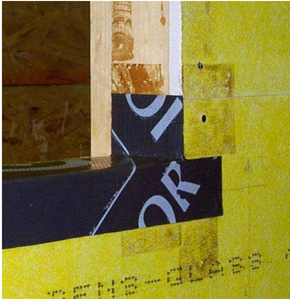
Figure 2.16. Rough opening treatment - Step 1. Figure 2.17. Rough opening treatment - Step 2.
