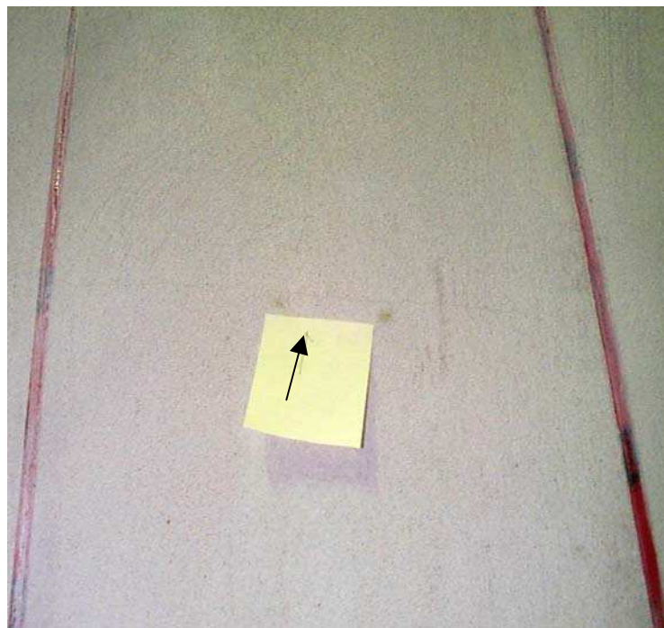
Figure 1.45. Crack between the vertical control joints (see arrow on sticker)
