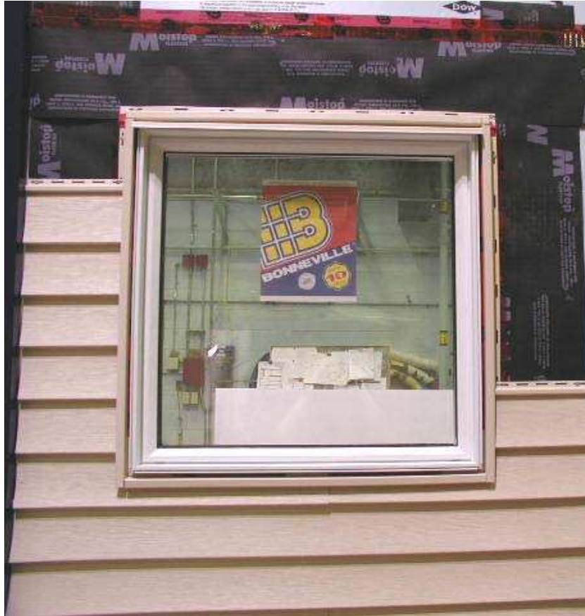
Figure A4.15 Specimen No.17. Installation of the vinyl siding and J-trim around the window frame
