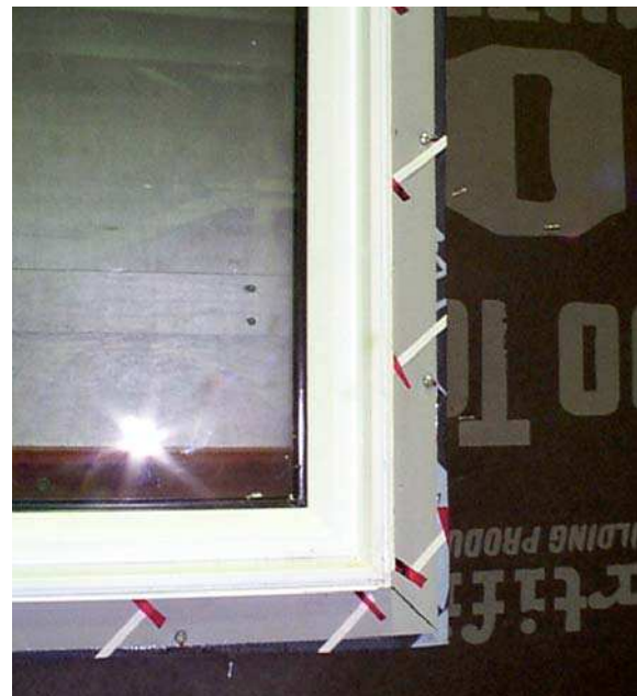
Figure 2.29. Wall No. 7. Deficiency: 6 mm gap between window flange and paper based WRB
