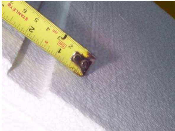
Figure 2.65. Wall No. 9. EPS insulation with vertical grooves, application of adhesive behind the insulation
