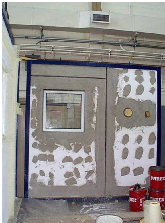
Figure 2.55. Wall No. 7. Spotting of fasteners and backwrapping completed
