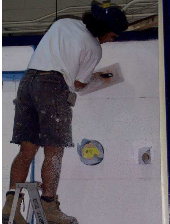
Figure 2.67. Wall No. 9. Sanding of EPS insulation
