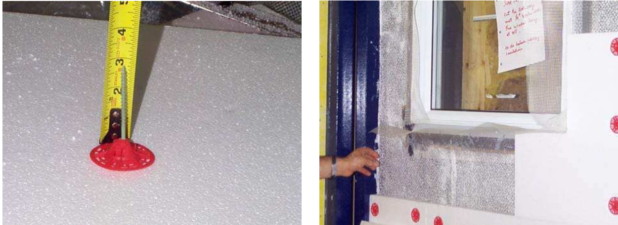
Figure 2.71. Wall No. 10. Rust proof fasteners and backwrapping over insulation
