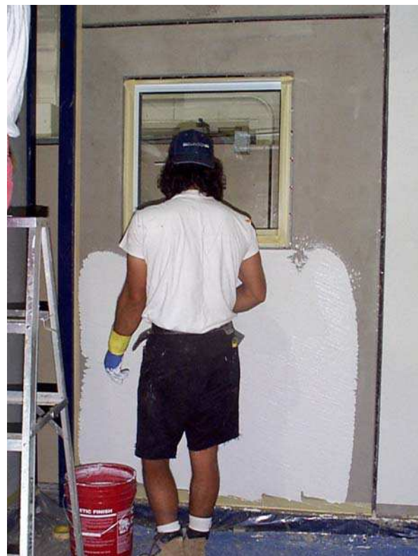
Figure 2.57. Wall No. 7. Application of finish coat
