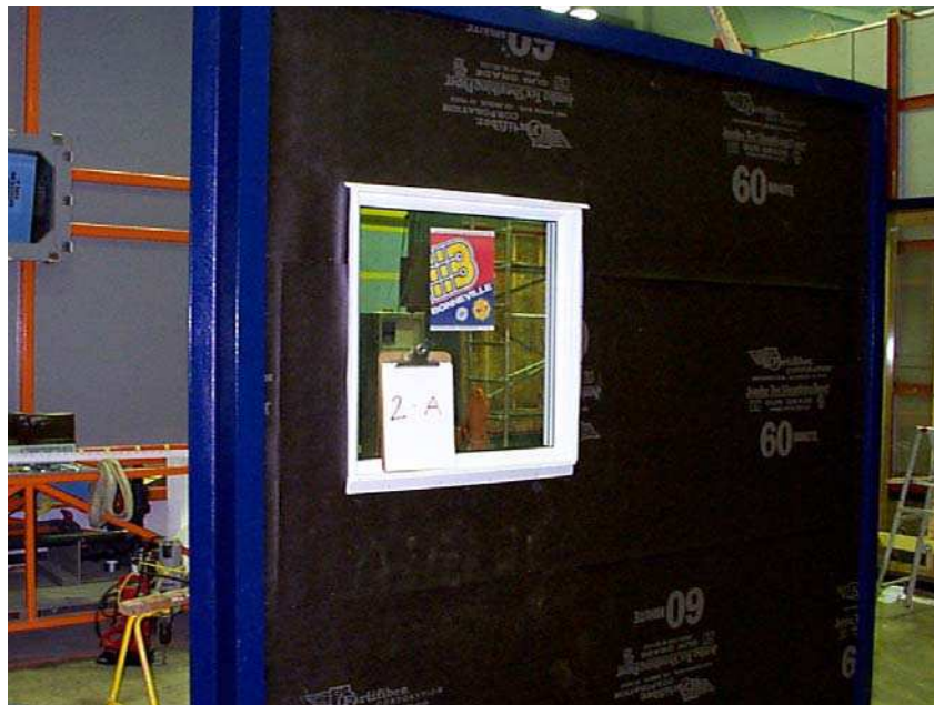
Figure 1.20. Window head elements in place before the last piece of paper-based water resistive barrier is applied
