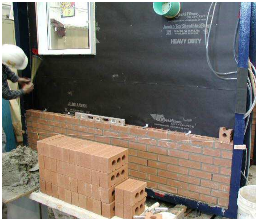
Figure A3.15 Brick laying in progress. Weepholes are placed every three bricks.
