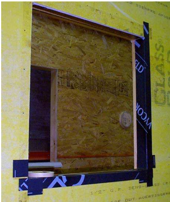
Figure 2.18. Rough opening treatment - Step 3. Figure 2.19. Rough opening treatment - Step 4.
