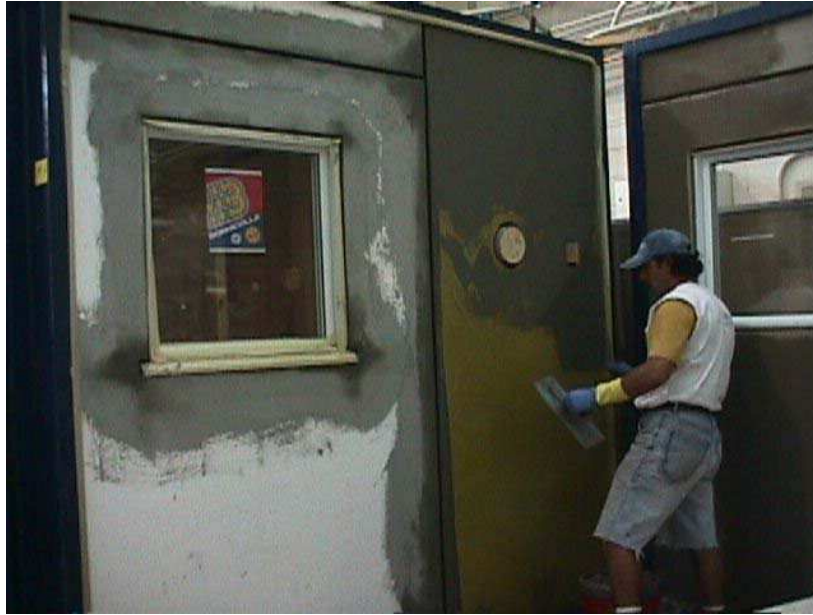
Figure 2.50. Wall No. 6. Application of mesh and base-coat
