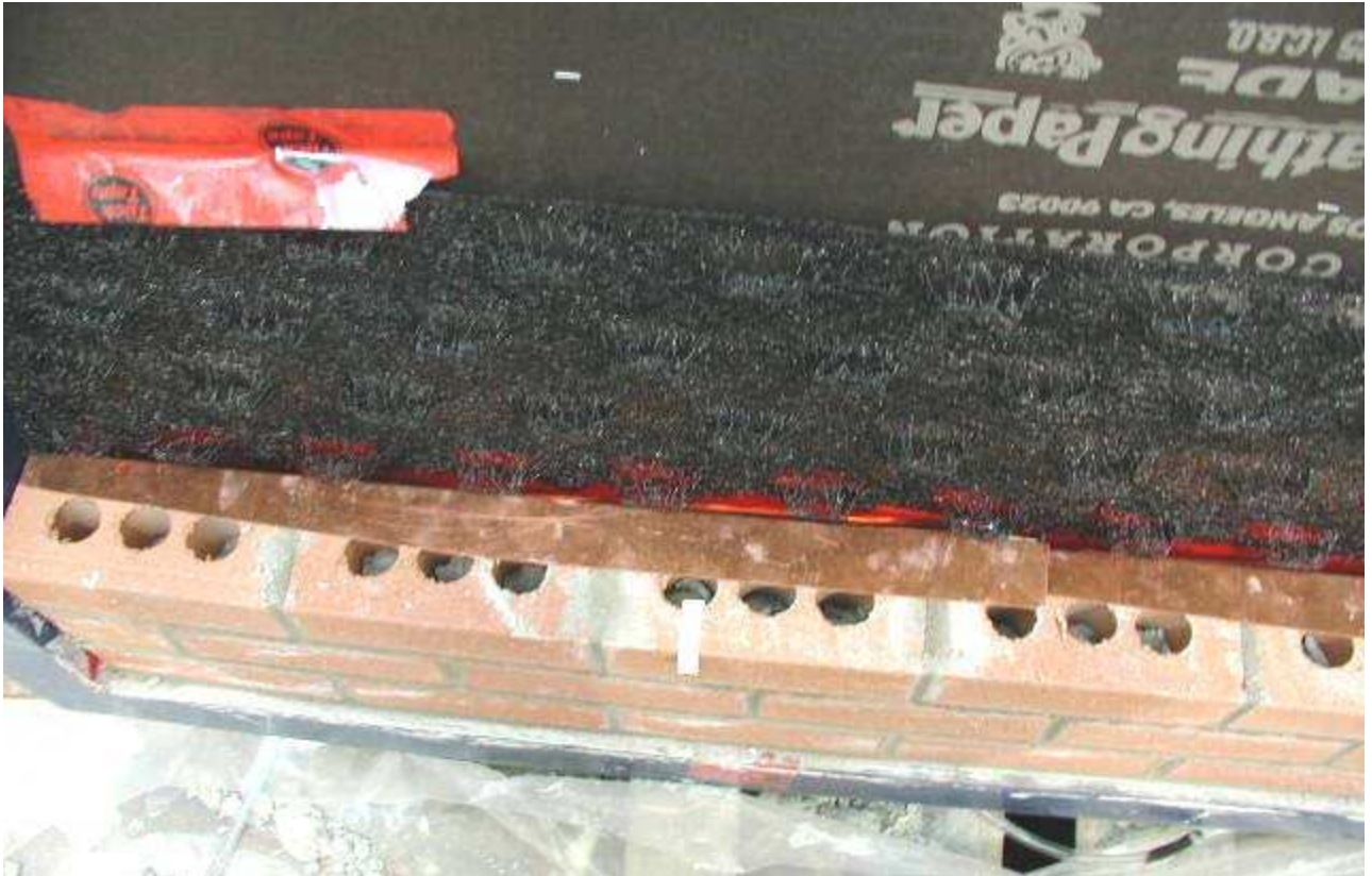
Figure A3.14 Descending view of the brick veneer. Mortar Maze was installed in the cavity to reduce the occurrence of mortar droppings in the water collection troughs.
