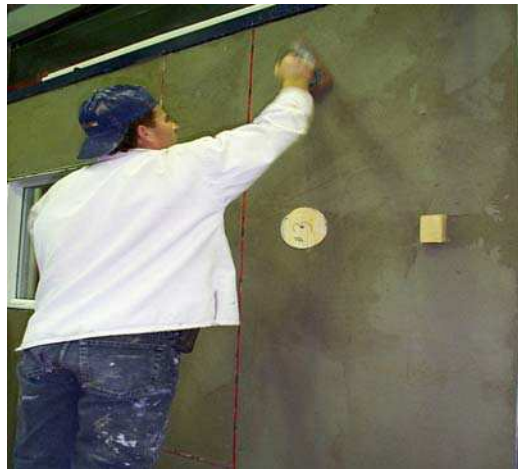
Figure 1.32. Floating of the brown coat on specimen No. 3
