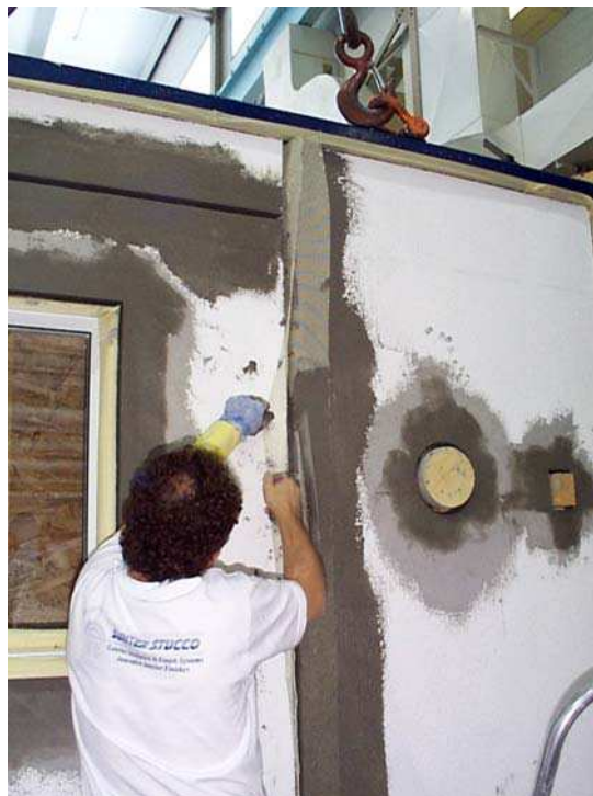
Figure 2.49. Wall No. 6. Backwrapping of EPS insulation
