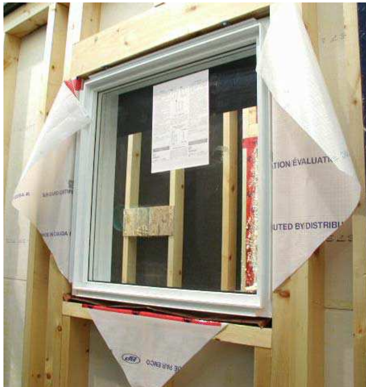
Figure A3.19 Installation of the window on specimen No. 14. Dupont procedure was followed.
