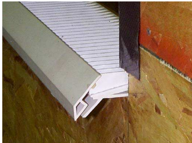
Figure 2.22. Front of prefabricated sill - Wall No. 6.
