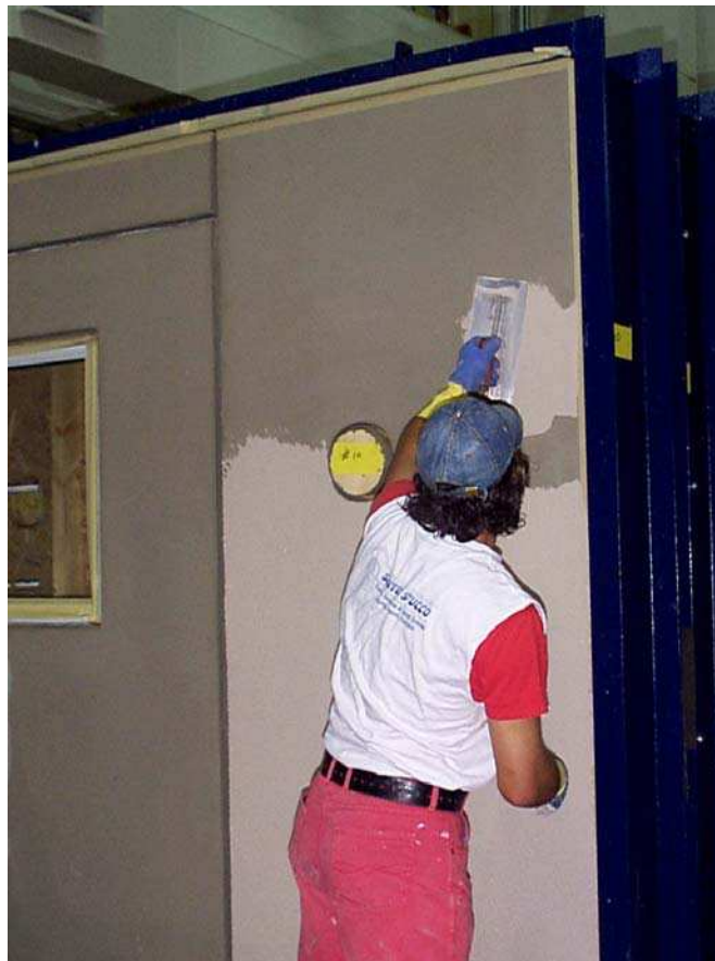
Figure 2.74. Wall No. 10. Application of finish coat
