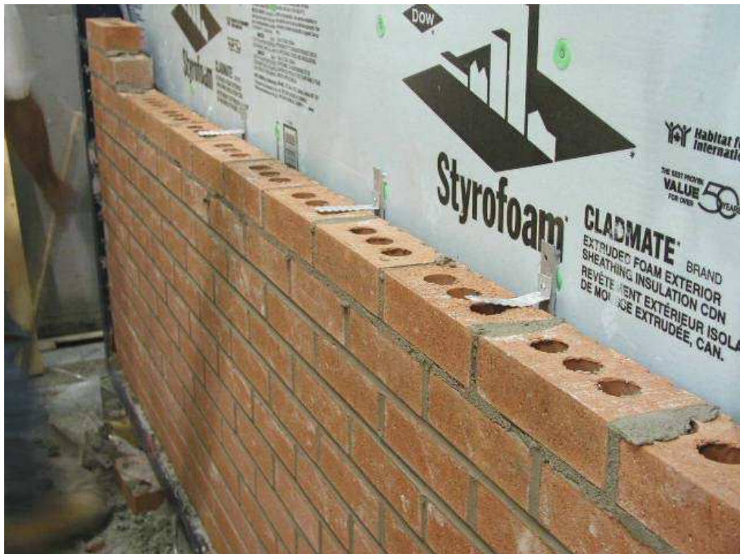
Figure A3.6 Specimen No. 11. Brick laying by a local masonry company
