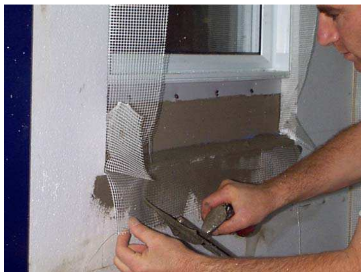
Figure 2.32. Backwrap for sill piece - Wall No. 8.
