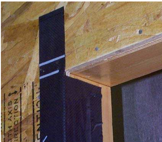
Figure 2.25. Deficiencies at top and bottom of jamb flashing membrane.
