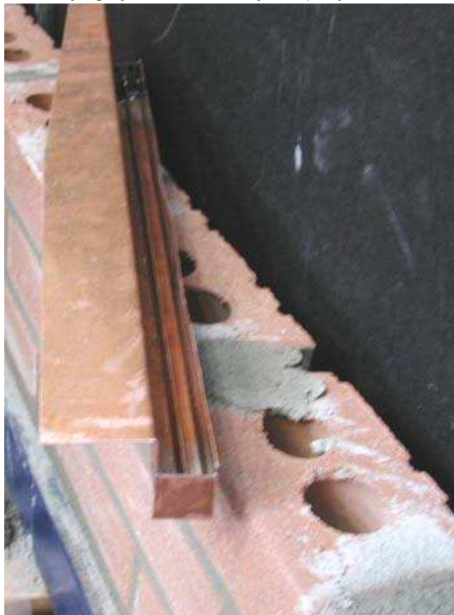
Figure A 3.7 Profile of a water collection trough to be placed in the cavity
