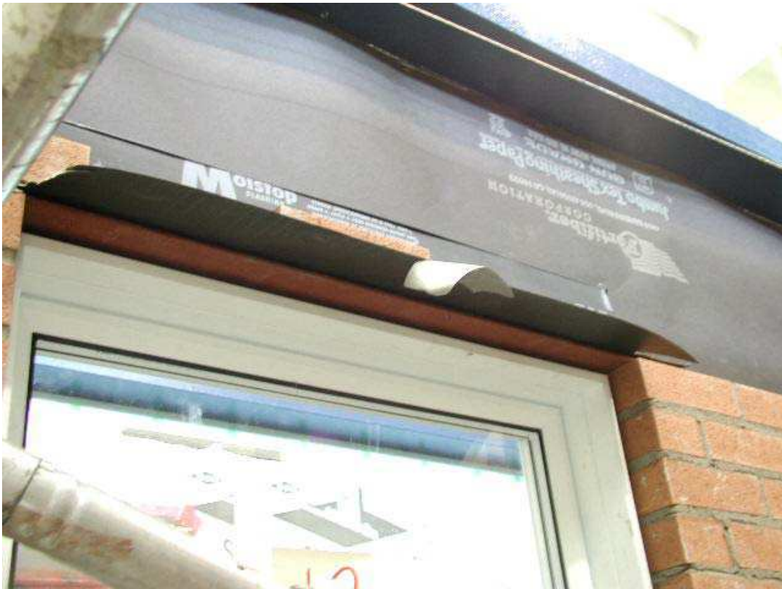
Figure A3.10 Specimen No. 12 at window head showing the shelf angle and the flashing membrane
