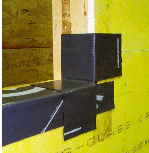
Figure 2.16. Rough opening treatment - Step 1. Figure 2.17. Rough opening treatment - Step 2.
