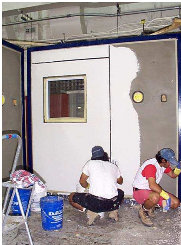
Figure 2.68. Wall No. 9. Application of finish coat
