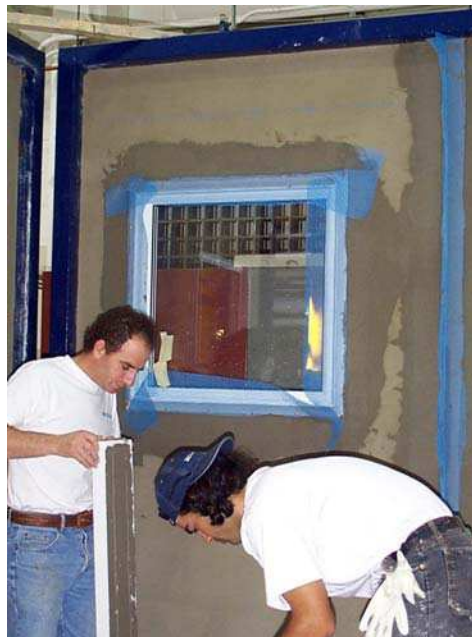
Figure 2.63. Wall No. 9. Backwrapping around openings
