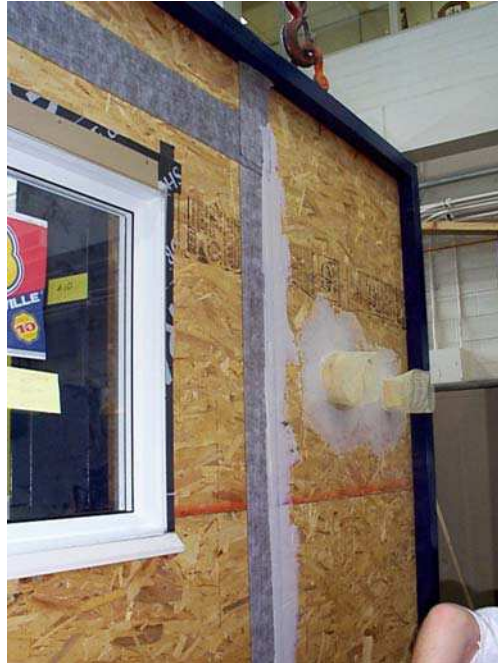
Figure 2.46. Wall No. 6. Self-adhesive membrane behind control joints and backwrapping of penetrations
