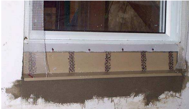
Figure 2.33. Sill drip flashing with drainage pieces - Wall No. 8.
