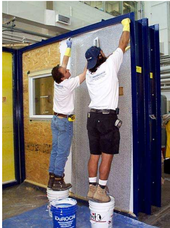
Figure 2.69. Wall No. 10. Application of WRB coating and nylon drainage mat
