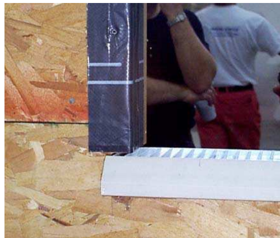
Figure 2.25. Deficiencies at top and bottom of jamb flashing membrane.
