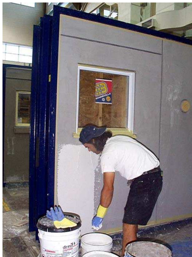
Figure 2.51. Wall No. 6. Application of finish coat
