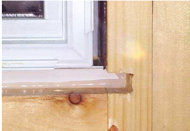
Figure 2.23. Prefabricated sill embedded in sealant - Wall No. 6.
