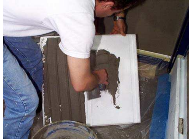
Figure 2.65. Wall No. 9. EPS insulation with vertical grooves, application of adhesive behind the insulation
