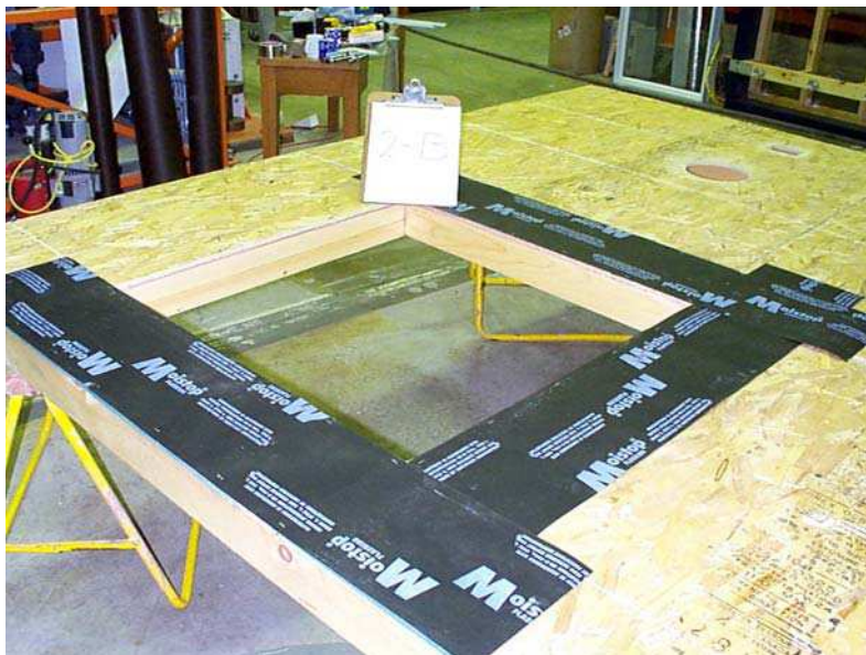
Figure 1.19. Installation of sill and jamb flashing on wall 2b
