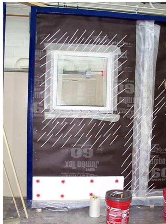
Figure 2.53. Wall No. 7. Backwrapping of vertical joint and insulation installation
