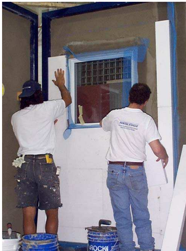
Figure 2.66. Wall No. 9. Installation of EPS installation
