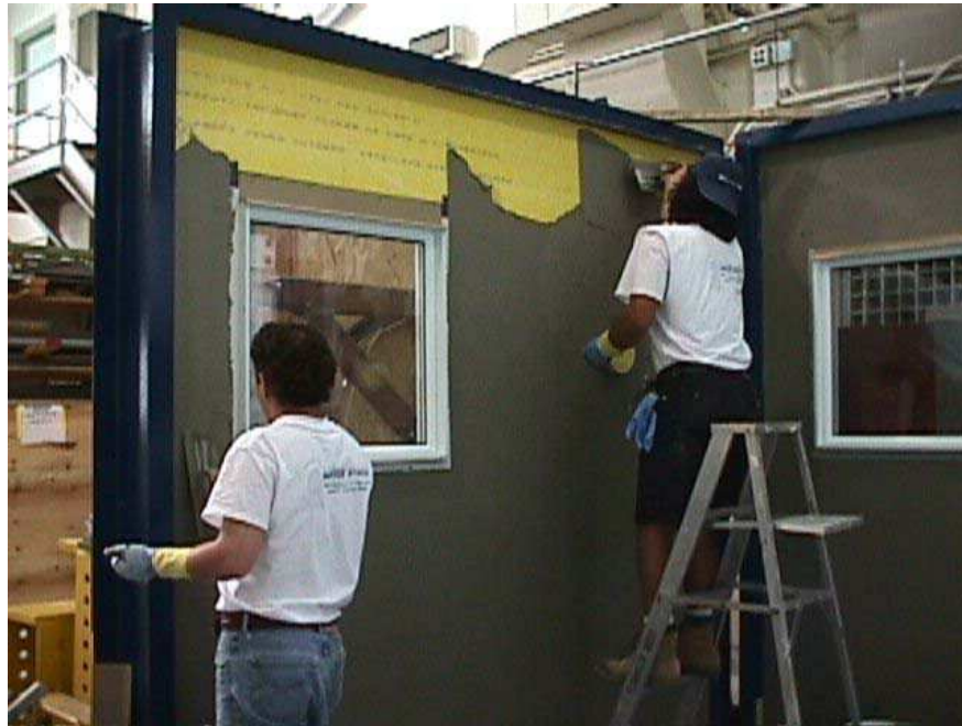
Figure 2.58. Wall No. 8. Application of WRB coating
