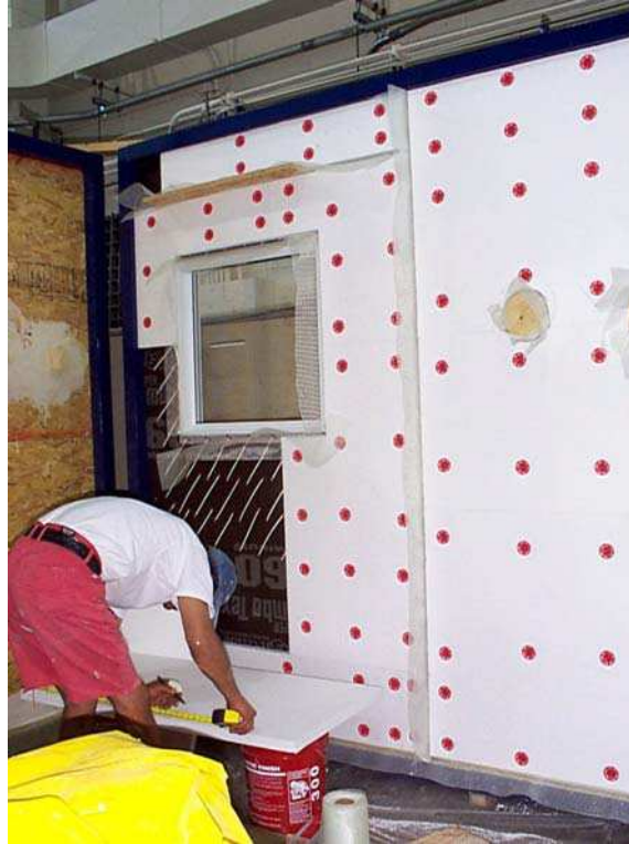
Figure 2.54. Wall No. 7. Insulation mechanically attached
