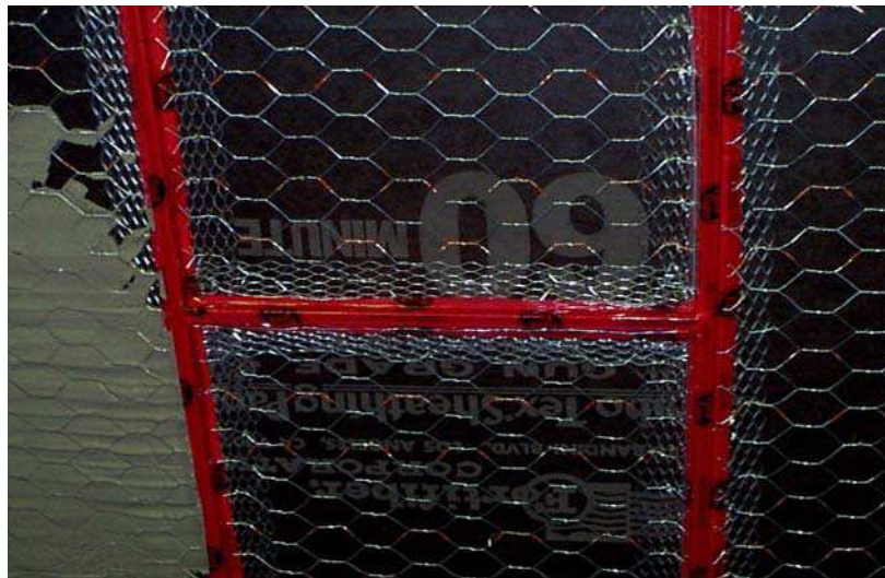
Figure 1.26. The control joints were covered with tape to reduce bonding of the stucco plaster to the metal control joint profile.
