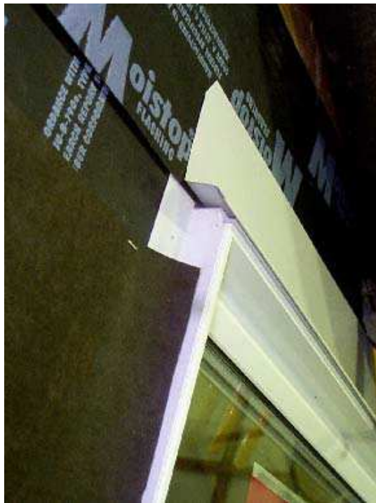
Figure 1.20. Window head elements in place before the last piece of paper-based water resistive barrier is applied
