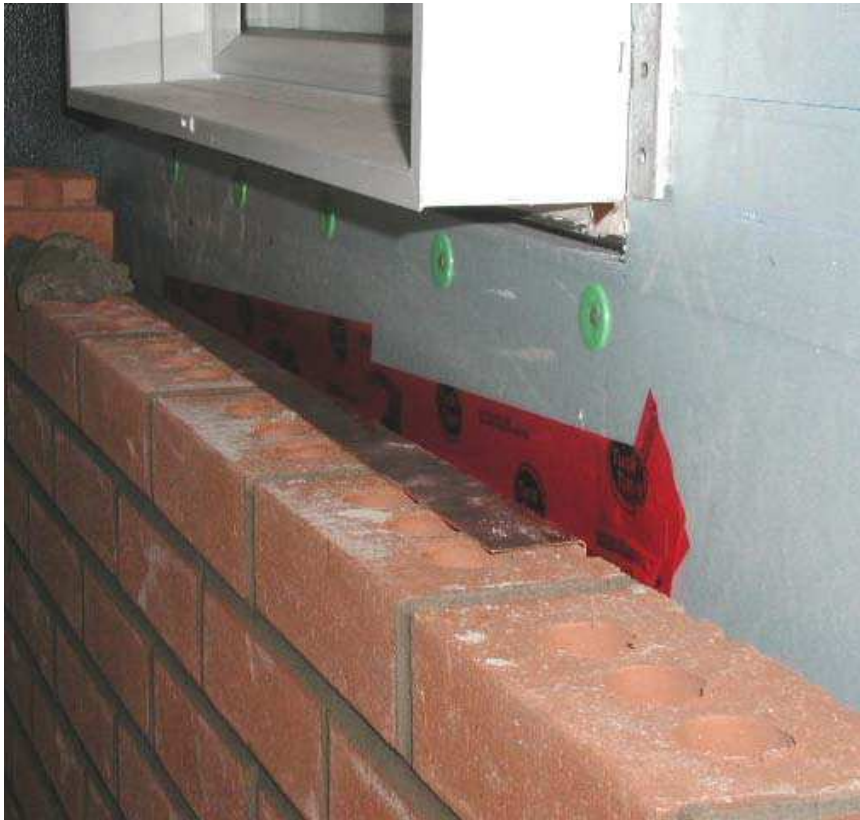
Figure A3.8 Window frame extension and installation of the water collection through in the cavity behind the brick veneer
