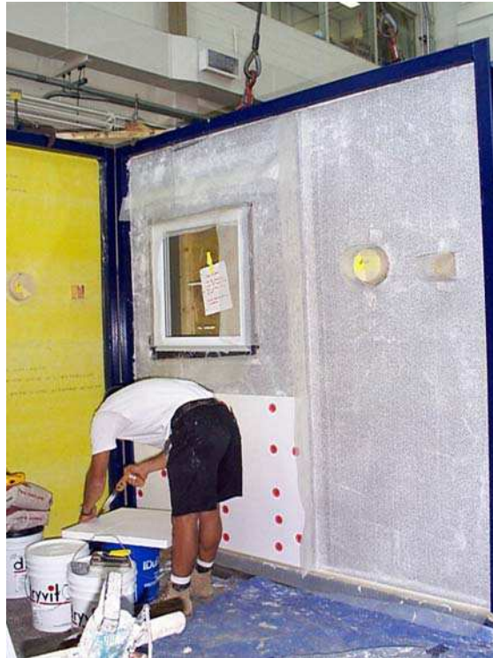
Figure 2.70. Wall No. 10. Installation of mechanically attached EPS insulation
