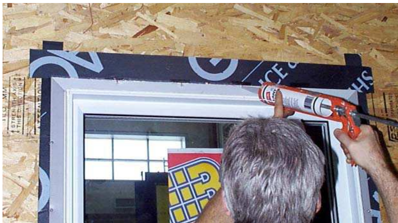
Figure 2.24. Sealant at top of jamb - Wall No. 6.
