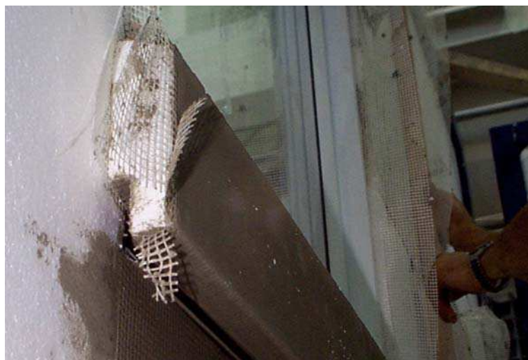
Figure 2.35. Sill piece installed - Wall No. 8.
