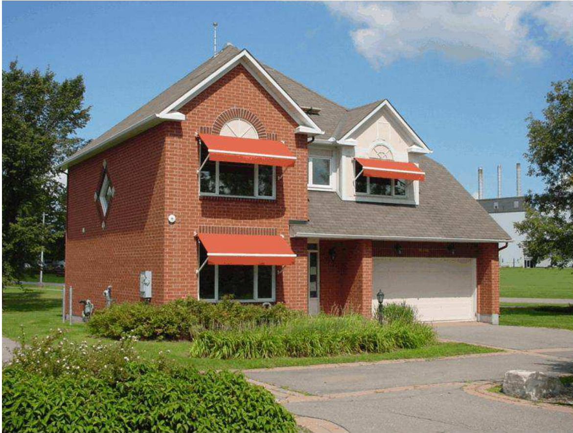
Figure 2. The Awnings on the Experimental House, photographed close to Solar Noon.
