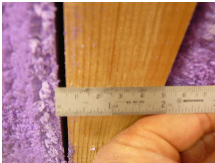
Figure 10 – Separation of SPF from framing due to higher than normal moisture content in studs. [1]
