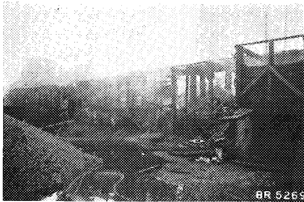
Fig. 7. Remains of coal dispersal chute after fire destroyed frame-covered section.
