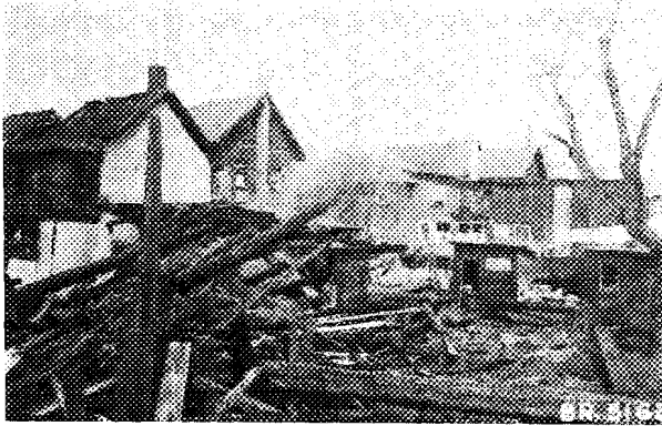
Fig. 4. Remains of wood frame warehouse. Note number of wood shingle roofs involved.
