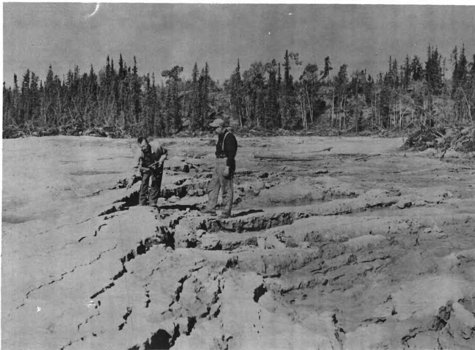
FIGURE 5 SILT EXPOSED BY REMOVAL of MUSKEG COVER SHOWING EFFECT of MELTING
