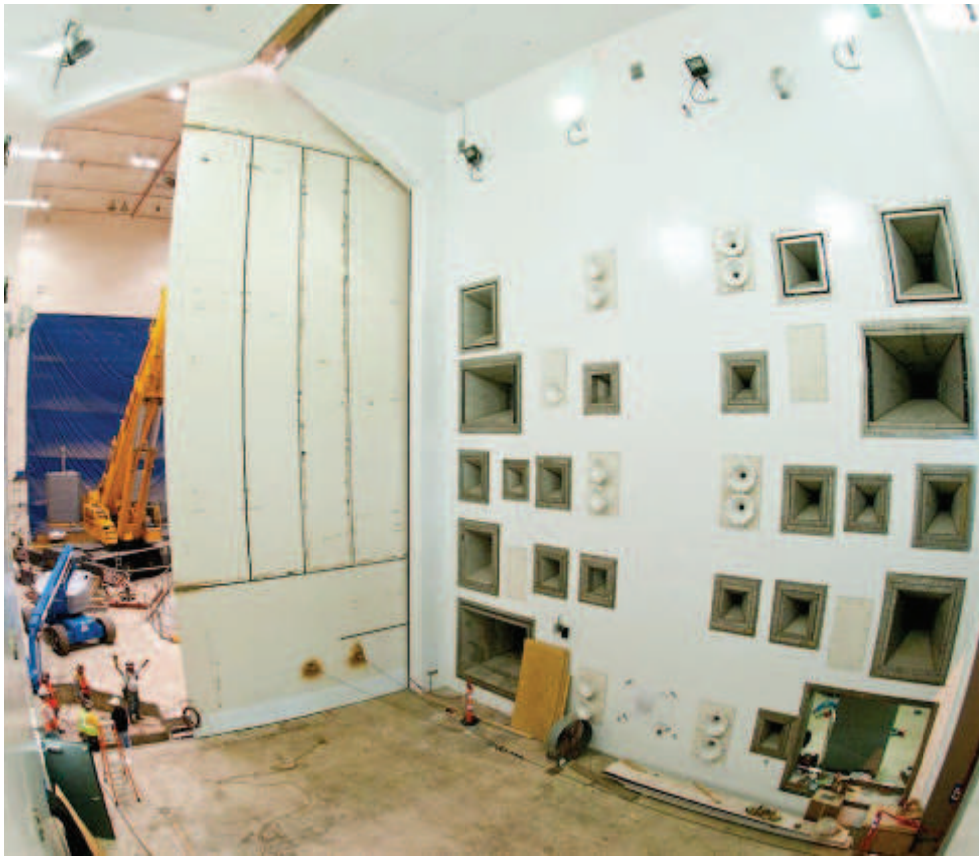
Figure 2: Ongoing Construction of the NASA Reverberant Acoustic Test Facility (RATF). The modulators are located behind the horn wall shown in the photograph.
