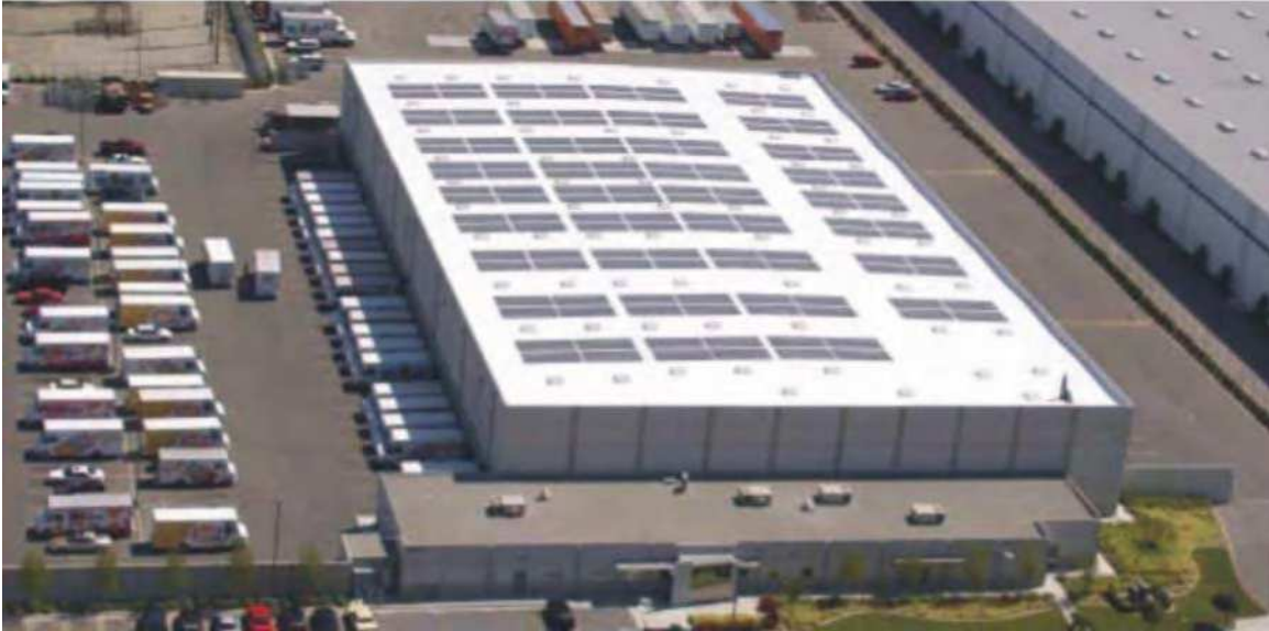
A solar electric roofing system (flexible photovoltaic [PV] modules laminated on thermoplastic membrane) is integrated into the Frito-Lay distribution facility in Los Angeles, Calif.
