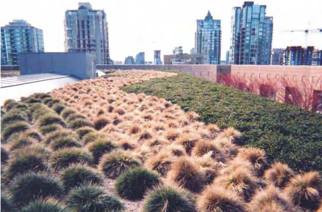
An intensive garden roof system (350-mm [14-in.] growing medium planted with ornamental grasses) on the rooftop of the Vancouver Public Library in B.C.
