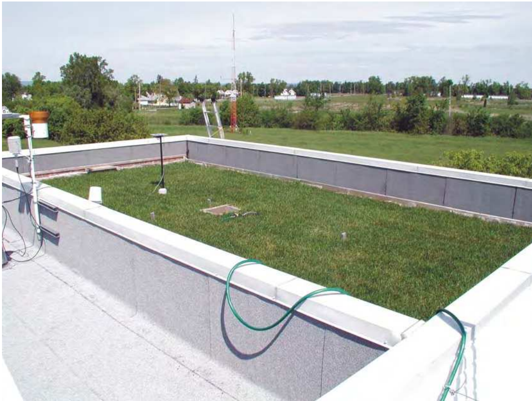
An extensive garden roof system (150-mm [6-in.] growing medium planted with grasses) on the National Research Council's (NRC's) Institute for Research in Construction (IRC) field roofing facility in Ottawa.
