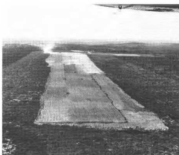
FIGURE 3. Air view to west of runway under construction, August 1957. Note small lake in foreground being back-filled; shadings on runway indicate different types of rock fill (shale, dolomite, quartzite) from quarry in distant background.
