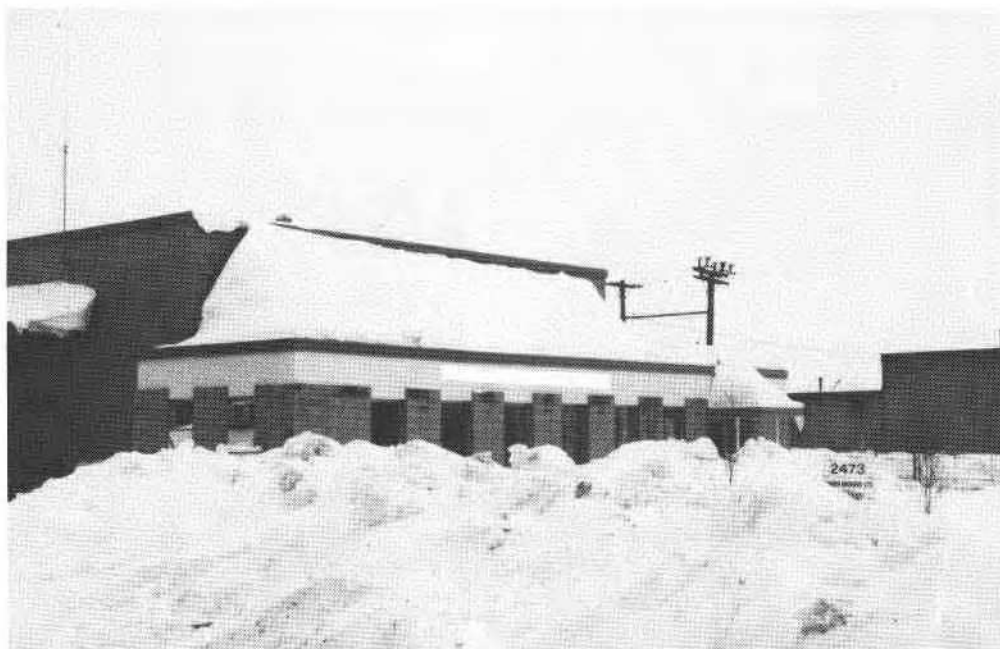
Fig. 16. Large "triangular" drift in the lee of the upper roof of Ottawa Sufferance, mid-January 1978 ( \Delta H/H = 0.48 ).
