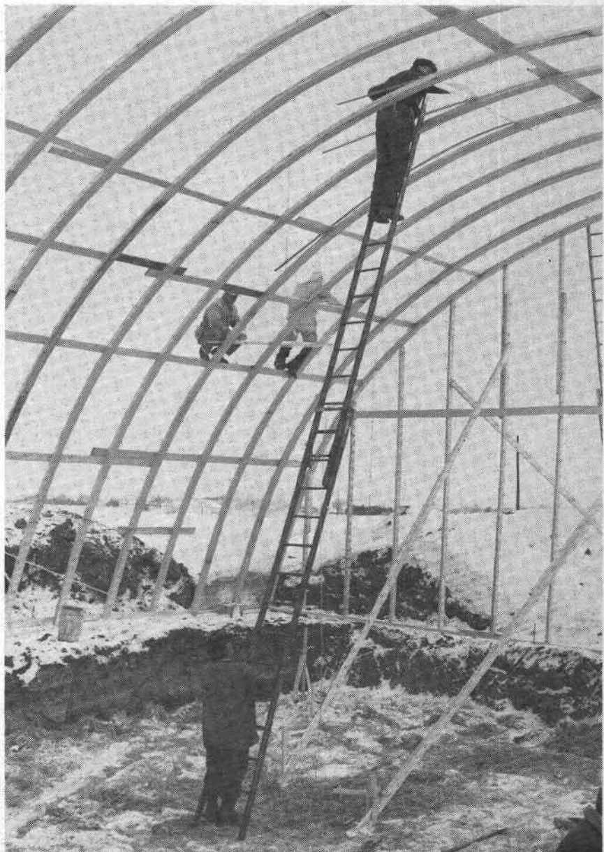
PLASTIC ROLLS 6 ft. wide were cut into 37 ft. lengths and re-rolled round a 6 ft. length of timber. End of the 37 ft. roll was tacked to ridge beam and then unrolled and tacked to arch ribs.
