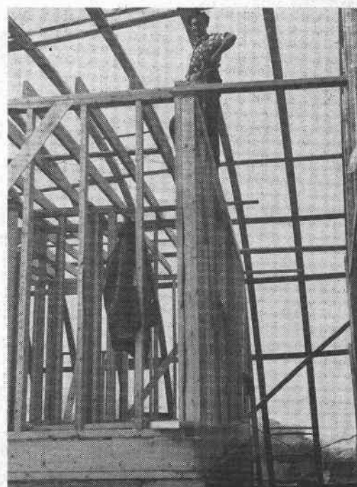
WORKING UNDER THE SHELTER with outside temperatures below freezing point, the tradesmen found conditions warm enough without special heating to move around in open-neck shirts with sleeves rolled up.
