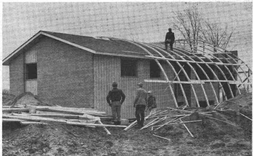
DISMANTLING THE SHELTER with the house closed in was simple. Two workmen in rubber boots stood on the roof and carried the disconnected arch ribs to the end of the house and lowered them to the ground.
