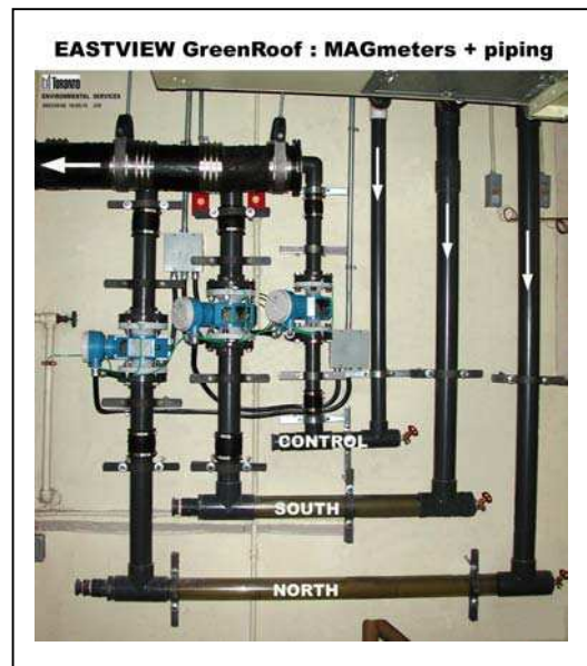
Figure 6 Piping and MAGmeter layout
