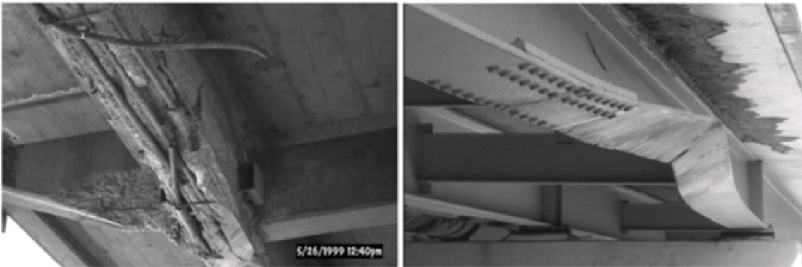
Figure 3: Damage to concrete and steel bridge girders resulting from overheight vehicular impacts (Sharma et al., 2008)
