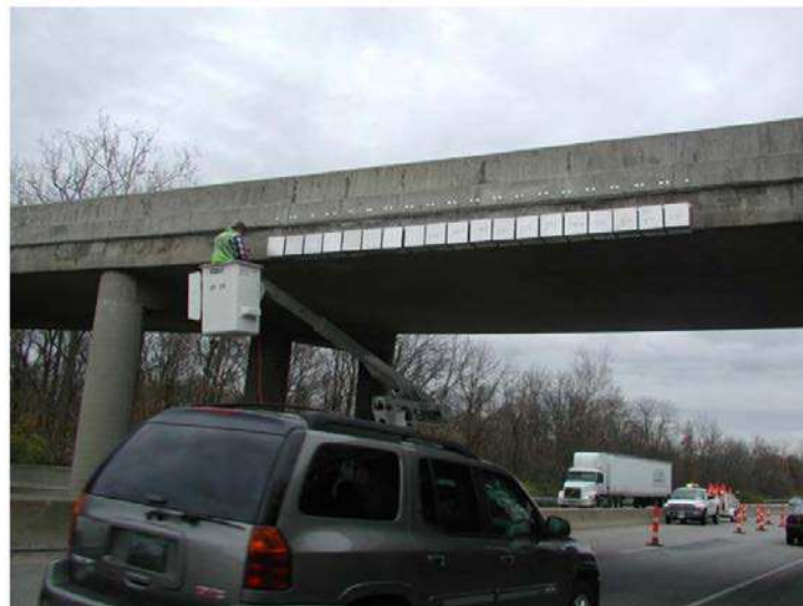
Figure 6: Field installation of I-Lam panels on concrete bridge (DEL-23-12.99) in Delaware, U.S. (Qiao et al., 2008)
