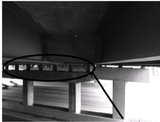
Figure 7: Bridge in Georgia elevated using steel pedestals (Hite et al., 2008)
