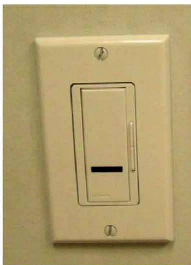
*Figure 6. Wall-mounted personal lighting controller at the college.*
