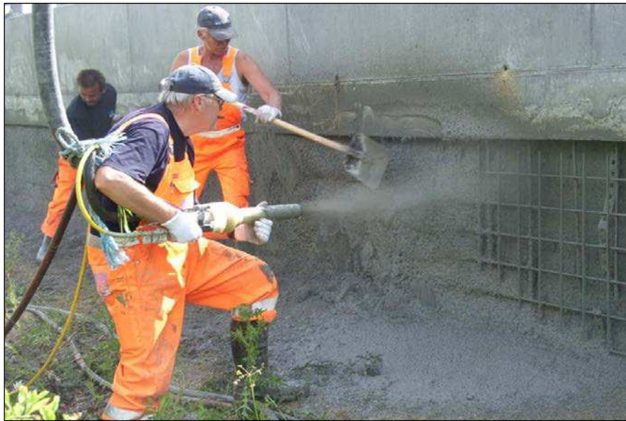
Fig. 10.3. Shotcreting of wall panels with SAP-modified concrete, Lyngby, Denmark [1].
