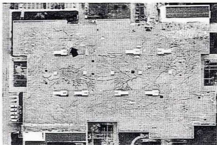
Figure 1 Aerial view of shattered ballasted unreinforced PVC roof system. Shatter initiated at the upper left, where indicated by the arrow. The shatter propagated in a counter-clockwise direction. One area at the top center portion of the roof did not initially shatter. However, it shattered a few days later. Membrane replacement is underway at the upper right and lower left corners.
