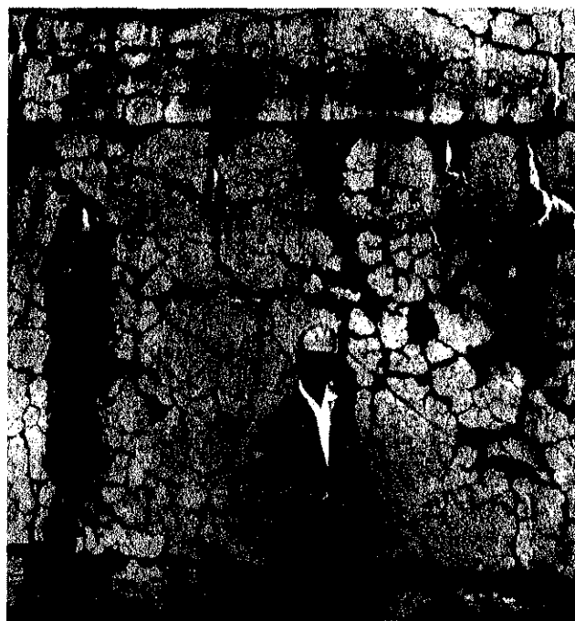
Fig. 1—Photograph of map-pattern cracking of retaining wall due to alkali-silica reaction at Canadian end of Saunders G.S.
