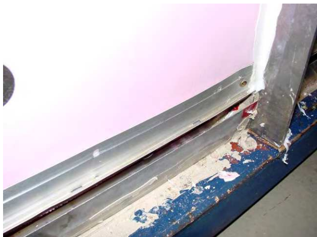
Figure 6 — Photos and related pictorials of collection troughs (a) trough for collection of water that drains from sill (b) trough for collection of water behind cladding at base of wall.
