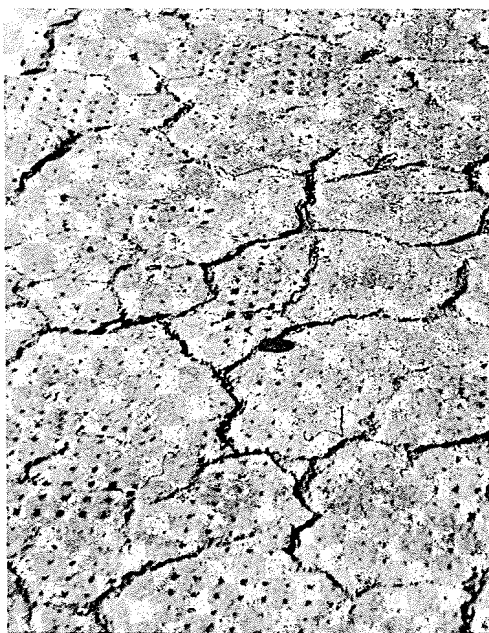
Figure 3. Typical pattern cracking in sidewalk in Kingston.
