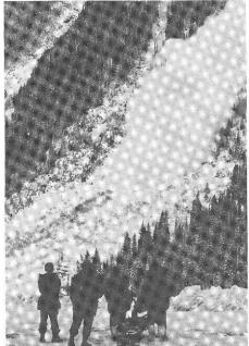
protection. Snowsheds, over which an avalanche can slide, protect troublesome sections of the Trans-Canada Highway in the Rogers Pass area. Because of the substantial cost, however (some \$10,000 a metre), their use is limited and road builders accept that there will be instances when a showshed is blocked off at the ends by a particularly large avalanche. After such an event the snow is simply cleared away with heavy equipment.
