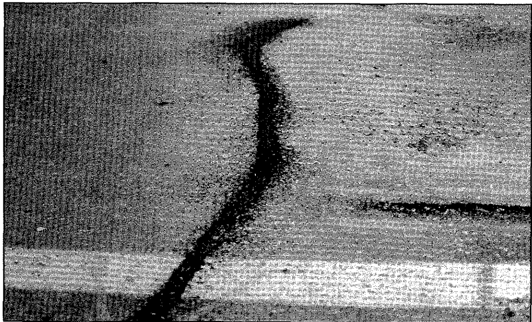
Figure 18. Typical blackening of an overheated rout
