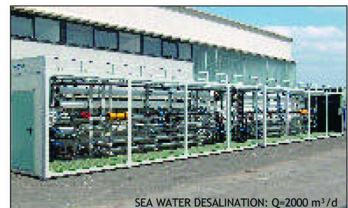
SEA WATER DESALINATION: Q=2000 \text{ m}^3/\text{d}
