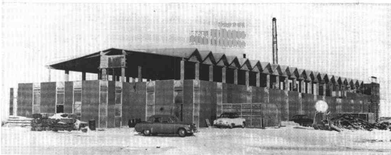
Fig. 2. Precast concrete roof and frame provide the structural portion of a lightweight enclosure (University of Saskatchewan).
