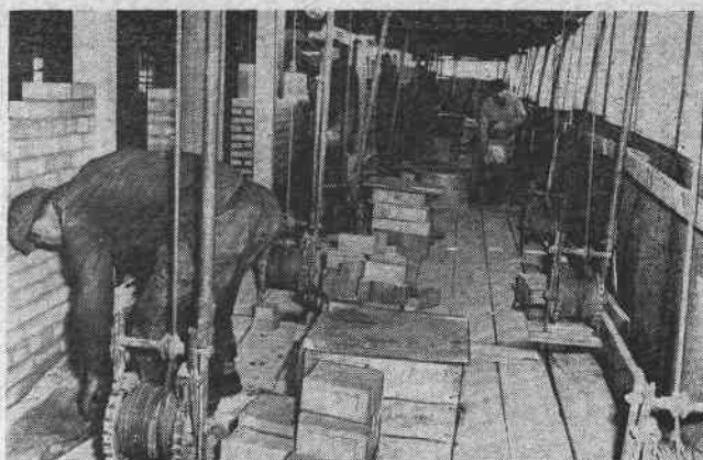
... AND HERE'S WHAT it looked like inside. Brickwork is going ahead many stories up with the men operating under near-ideal conditions despite severe weather outside. (Illustration 6.)
