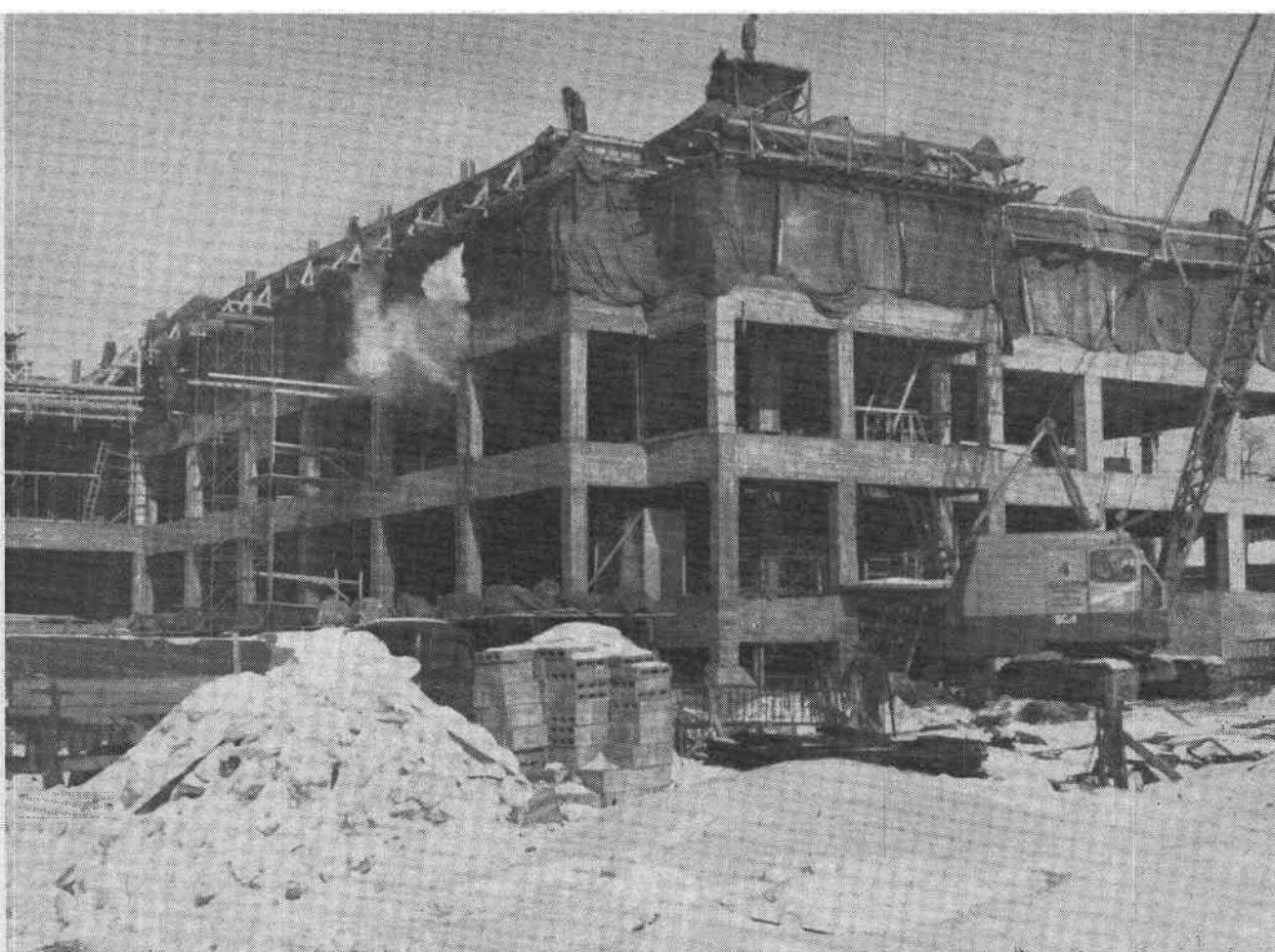
HERE'S A GOOD EXAMPLE showing that building under a winter enclosure can be carried out in all sizes of projects. This is the new Survey and Mapping Building in Ottawa using an upper floor enclosure of timber forms and hanging tarps. Top surface of the roof slabs is covered with an insulating blanket. (Illustration 10)
