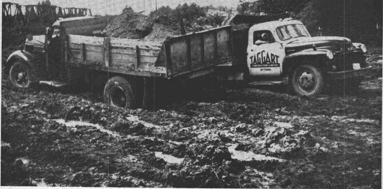
ANOTHER SUMMER BUILDING HAZARD. This also happened in Ottawa after rain in summer when transport became bogged down around a job-site. It could seldom happen in winter when the ground would be frozen. (Illustration 2).
