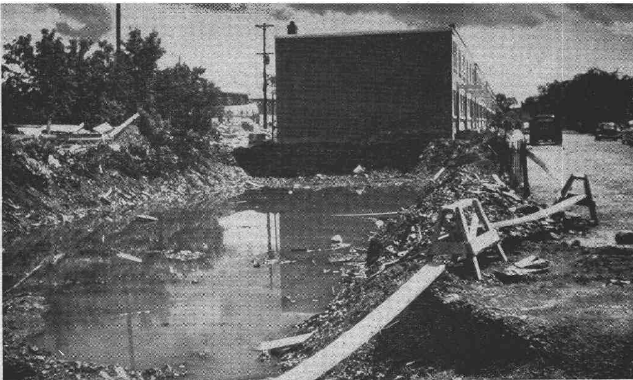
SUMMER BUILDING ALSO HAS ITS HAZARDS. Here time was lost and extra costs were incurred in this apartment summer-building project in Ottawa when the flooded excavation had to be pumped out after rain. (Illustration 1).
