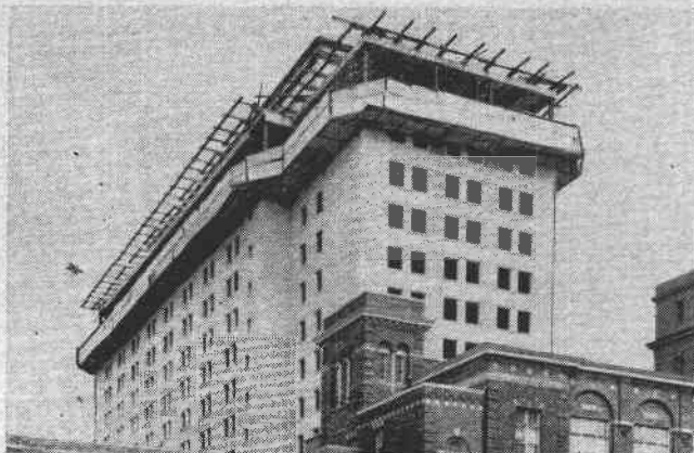
COVERED-IN SUSPENDED SCAFFOLD. This covered scaffold, enclosing a story-high stage of construction, was used in Toronto. It is raised as the work proceeds. (Illustration 6.)
