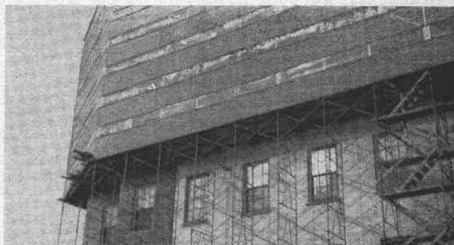
... AND HERE IS ANOTHER method for enclosing multi-story buildings, also from Halifax. It is the Maritime Telephone and Telegraph Building where standard scaffolding was braced against the building frame. (Illustration 7.)
