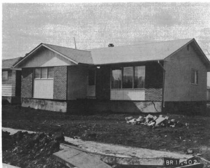
Fig. 2 Thawing of permafrost has caused house foundation to settle unevenly.
