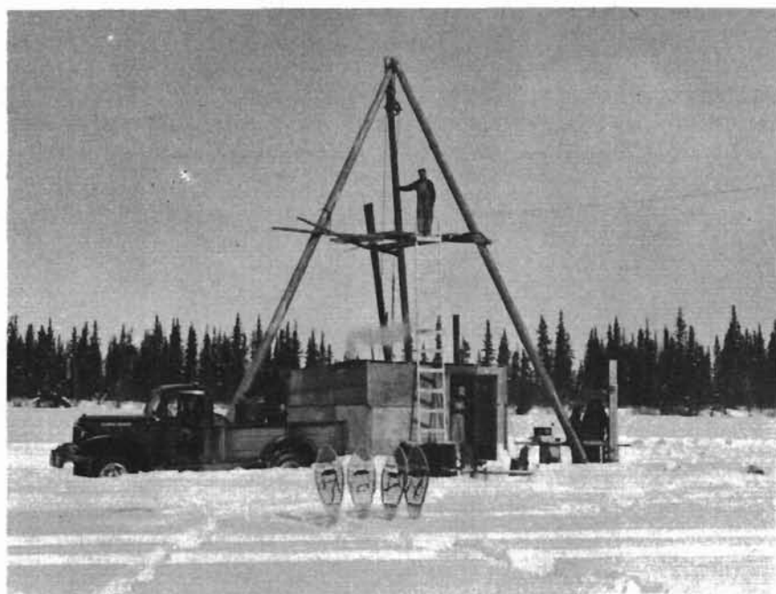
Fig. 4 Drill set-up at Hole No. 1 (centre of lake). Note core sampling table to right of drill shack and depth of snow cover.
