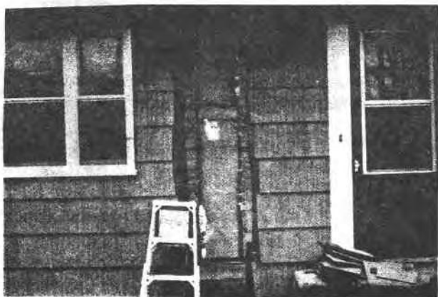
FIG. 2—Case I. Wood sheathing removed from one stud space. Batts now flush against the sheathing. UF foam not visible. Note curvature of paper-enveloping membrane on the batt at the sides of the cavity.
