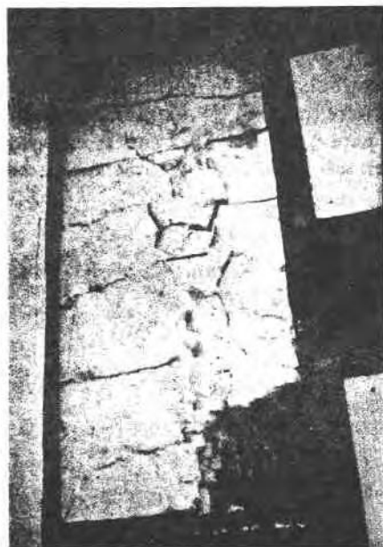
FIG. 14—Case III. Closer view of top stud cavity. Note extensive cracking in the foam caused by the compressed insulation batt pressing the foam against the outer wall, thus restricting movement.
