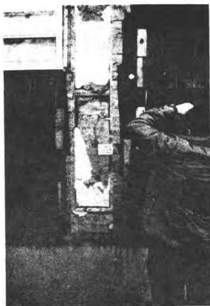
FIG. 11—Case II. North wall, sheathing removed, showing the UF foam partially filling the air space and partially filling the batt.
