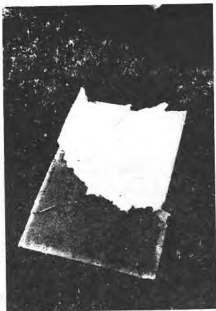
FIG. 15—Case III. The stud cavity immediately below the previous cavity. Note the outline of where the foam had been installed against the bag.
