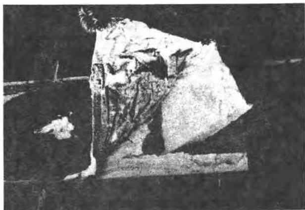
FIG. 8.—Case II. UF foam installed between the vapor barrier and the interior gypsum wallboard.
