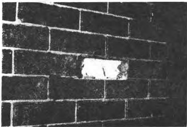
FIG. 18—Case IV. UF foam damaged by removal of the brick.
