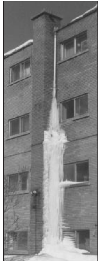
Figure 12. Severe icing below break in downspout
