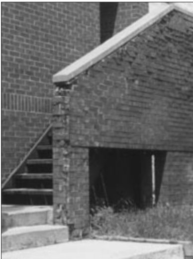
Figure 1. Frost damage (coping allows water to drain onto the wall)
