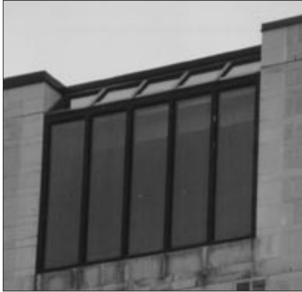
Figure 5. Staining below window (no sill projecting beyond wall)
