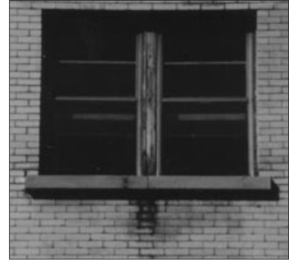
Figure 7. Staining beneath junction in a window sill
