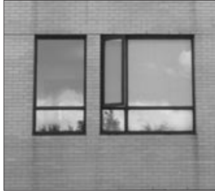
Figure 6. Staining below windows (no end barriers on sills)
