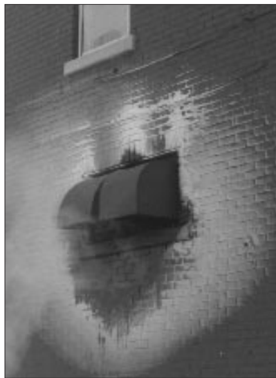
Figure 11. Frost on wall at a laundry exhaust vent
