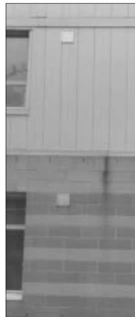
Figure 9. Staining below junction in flashing set back from the wall
