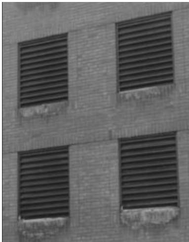
Figure 4. Staining and icing below garage vents (sills flush with the wall)
