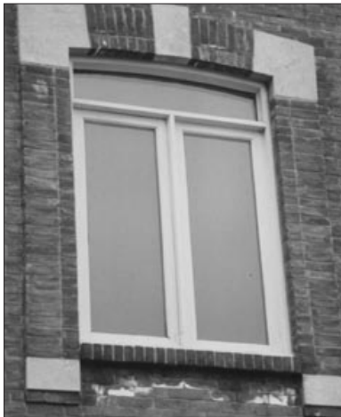
Figure 3. Efflorescence (water migrates through brick sill)
