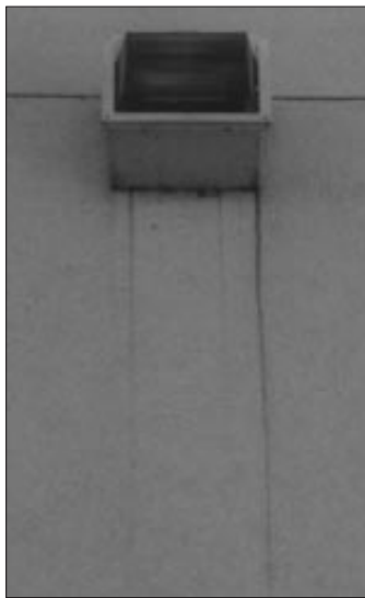
Figure 10. Staining below light fixture (water run-off)
