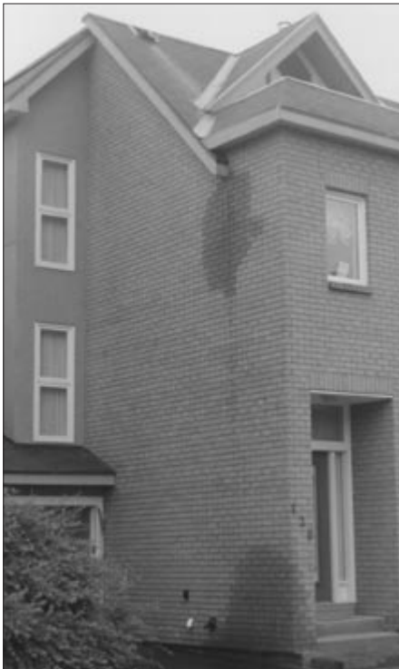
Figure 8. Wetting of wall from roof run-off
