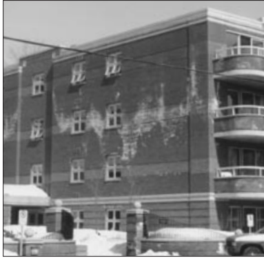
Figure 2. Efflorescence (coping allows water to drain onto the wall)
