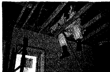
Insulation foam being sprayed inside the walls.
