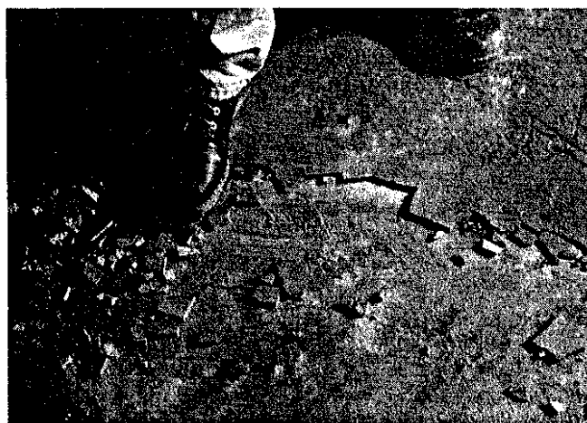
Fig 9 Crumbling of weak underlayment
