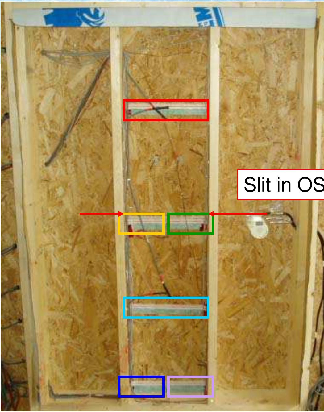
Diagram for Moisture Detection Tape Locations on the interior of the OSB
