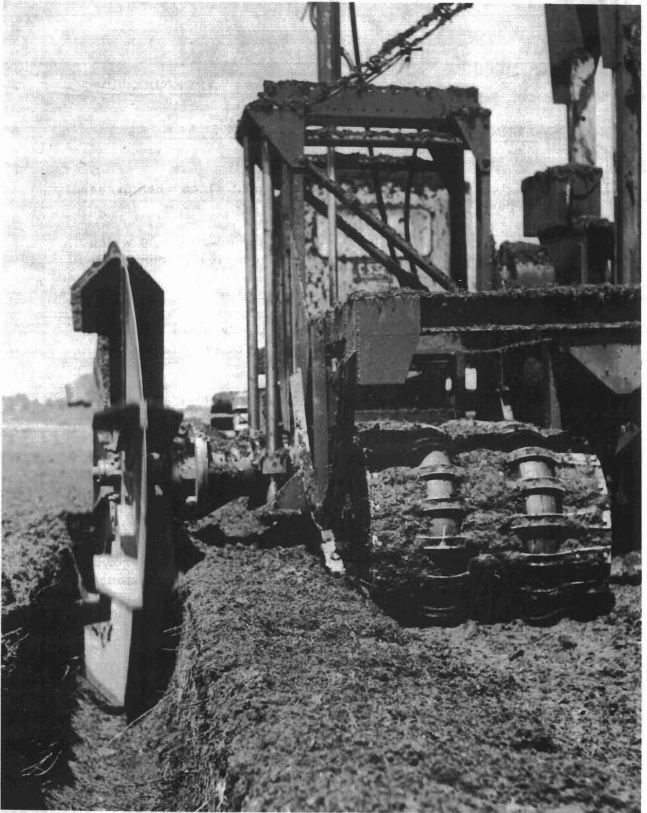
FIGURE 7 DRAINAGE DITCH EXCAVATED BY ROTARY DITCHER
